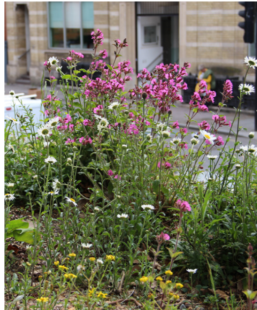
An extensive green roof with dry meadow plants in London Photo: Maria Ignatieva 2015
