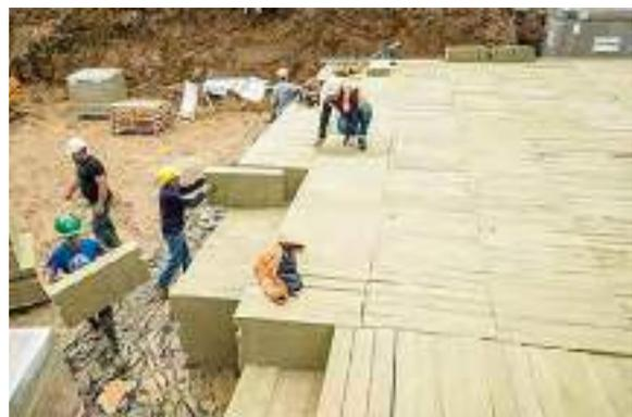
Originated from building insulation techniques, rockwool also has high absorption qualities. Due to its substantial amount of hollow space (up to 95%) combined with considerable constructive strength, it can be very effective as an immediate storage facility underneath porous surfaces. It is available on the market under a trademark of 'Lapinus'.
