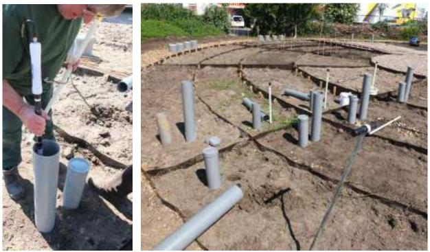
Installation of the hydrological monitoring pipes and the digital water loggers
