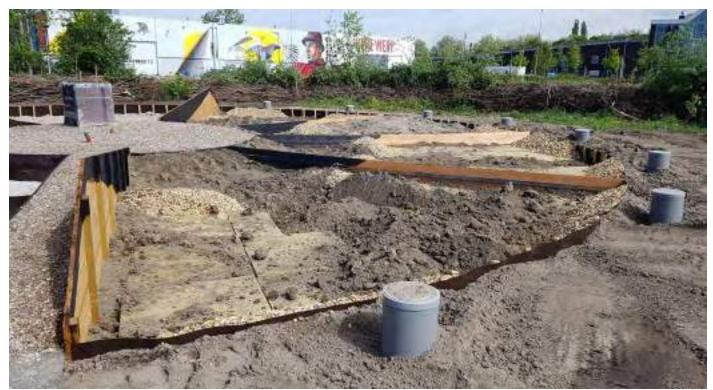
Shaping lower parts of bioswale and bringing diverse soil mixtures for mounds
