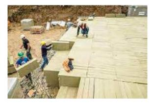
Originated from building insulation techniques, rockwool also has high absorption qualities. Due to its substantial amount of hollow space (up to 95%) combined with considerable constructive strength, it can be very effective as an immediate storage facility underneath porous surfaces. It is available on the marker under a trademark of 'Lapinus'.
