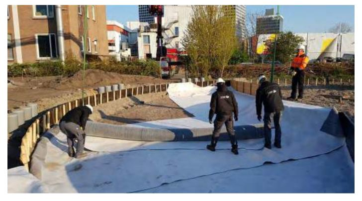
Separating various soils to allow monitoring - installing root shields, drainage pipes and a gravel layer
