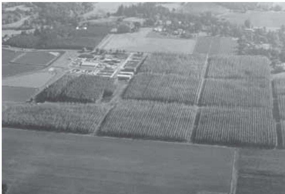
Fig. 6.32. Aerial view of the City of Woodburn, Oregon, USA, hybrid poplar stands used for treating municipal wastewater. Photo courtesy of J. Johnson.
