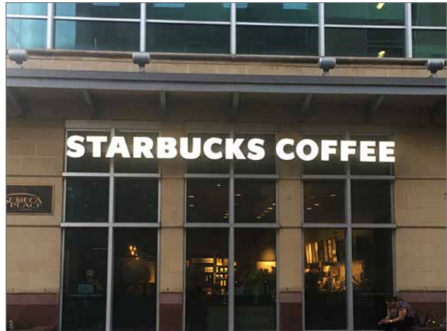
Figure 4.11 B. Example of an Internally Illuminated Letter Sign.
