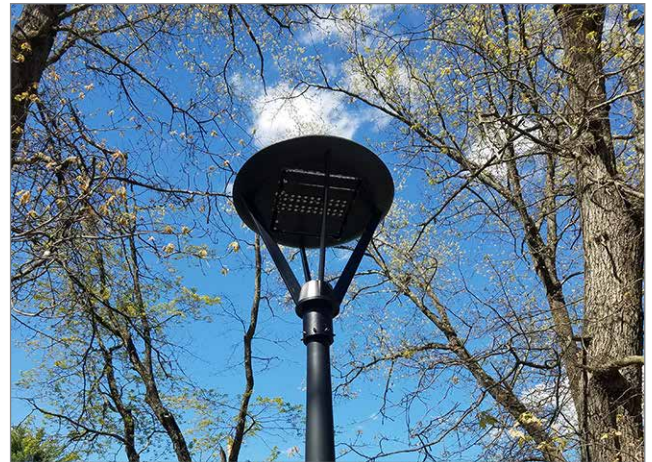
Figure 4.12 D. Example of an LED Solar Light.
