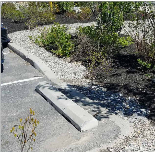
Figure 4.8 B. Bioswale with Dropped Curb Inlet.
