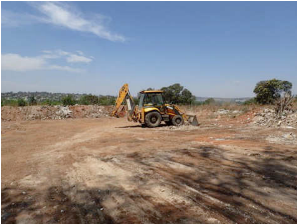
Figure 4 Cleared ground (rubble) with a TLB in the foreground
