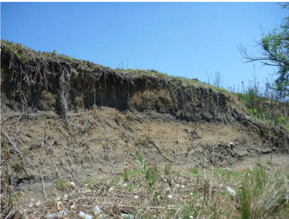
Figure 34 Eroded bank of the Jukskei River exhibiting soils that formed under uneroded valley bottom conditions
