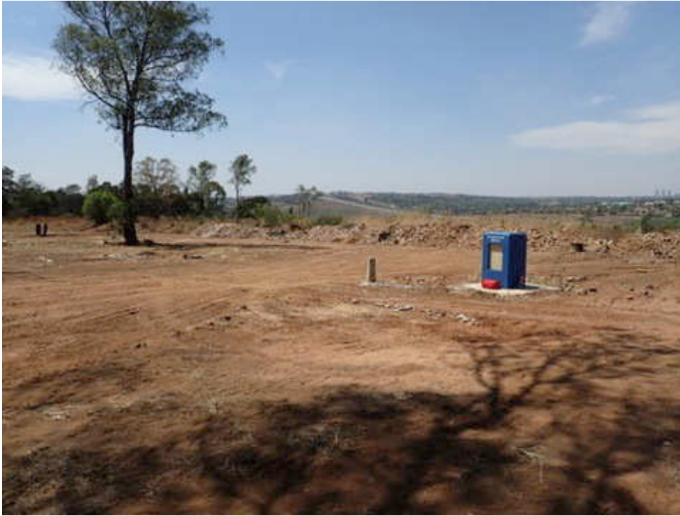
Figure 3 Cleared ground (rubble) with Rand Water pipeline markers
