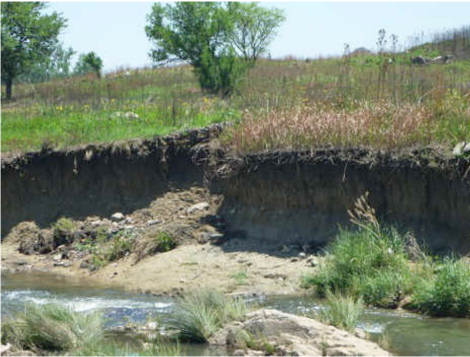
Figure 35 Eroded bank of the Jukskei River exhibiting soils that formed under uneroded valley bottom conditions. Note the wetland vegetation on the remaining bank.
