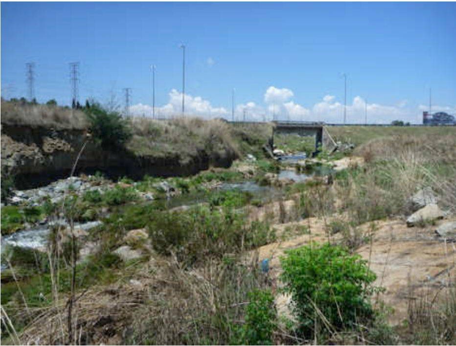
Figure 37 Eroded bank of the Jukskei River as a result of human activities
