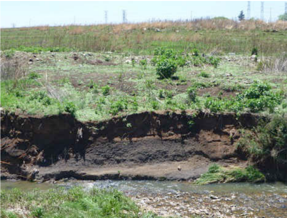
Figure 33 Eroded bank of the Jukskei River exhibiting soils that formed under uneroded valley bottom conditions
