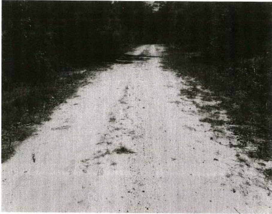
Photograph 7 – View of section of Brewers Road.
