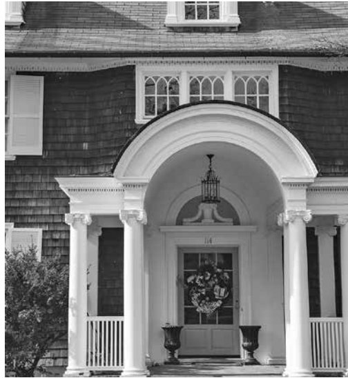
Creosote applied to cedar shakes produced the dark brown houses once universal in the neighborhood. Photo: Sally Foster
