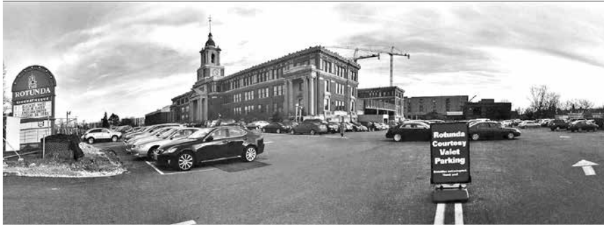
Mid-way through the construction. Photo courtesy of Hekemian & Co.
