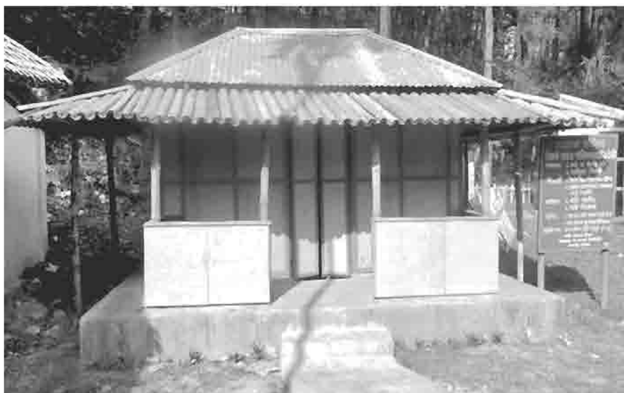
Figure 1. Model house-made of Cement bonded Particle Board
