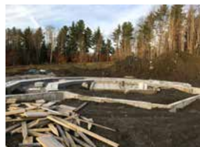
Strawbale home under construction.
