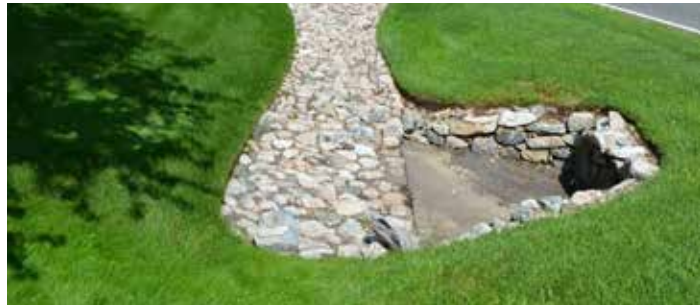
Culvert Sediment Catchment Basin with Riprap
