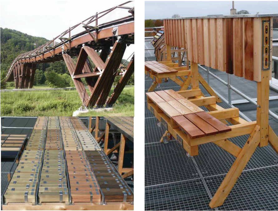
Fig. 2. Left top: Moisture monitoring on a timber bridge. Left bottom: MC recording on sandwich specimens made from modified and preservative treated timber. Right: Instrumented facade deck elements to quantify the effect of climatic changes on the moisture load of timber structures exposed at various locations in Europe
