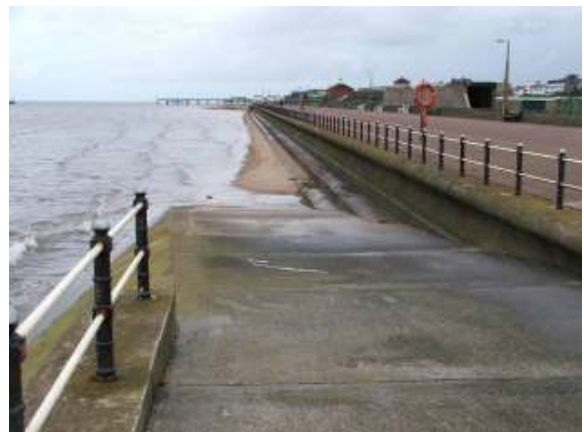
sea wall around Pleasure Island complex
