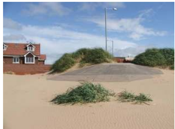
concrete revetment sea defence (opposite Todmorden Road) in St Anne's Dunes
