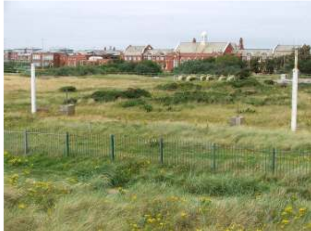
United Utilities pumping station, Fairhaven
