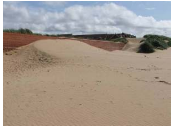
North Beach car park wall with accumulated sand
