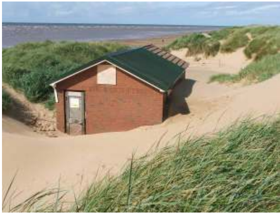
United Utilities pumping station (opposite Bentnick Road), St Anne's Dunes
