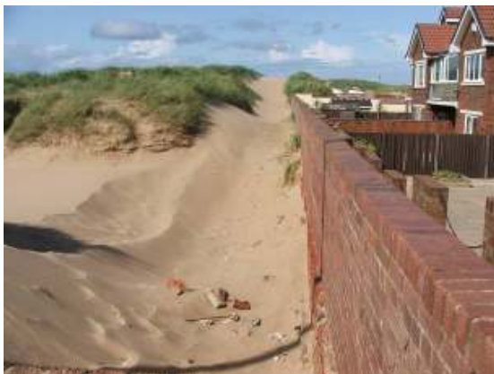
brick wall 'sea-defence' between beach and adjacent houses
