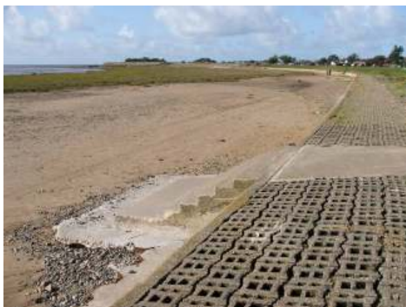
sea wall at top of Granny's Bay
