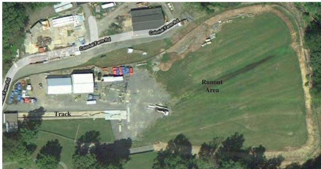
Figure 6.1. Aerial view of the FHWA FOIL facility.
