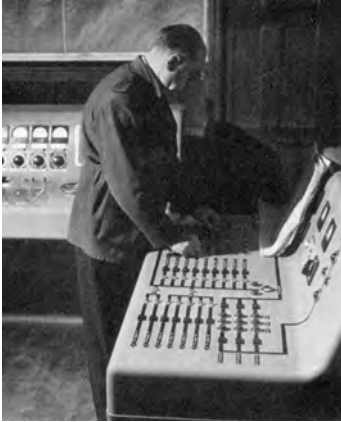
Fig. 2.23: Philips control desks for audio (left) and lighting. Fig. 2.24: Ground plan of light and sound installation for the 1954 spectacle “Les Féeries Nocturnes” at the château in Azay-le-Rideau.
