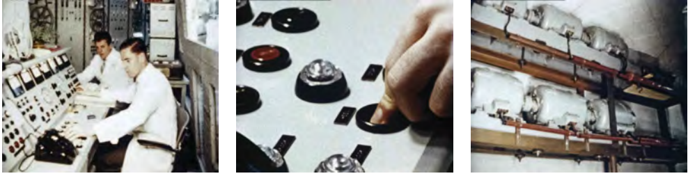
Fig. 2.93, 2.94 and 2.95: Wiel Cox at the central control desk (left); the button on the control desk that turned on the entire show (middle); the interlock system.
