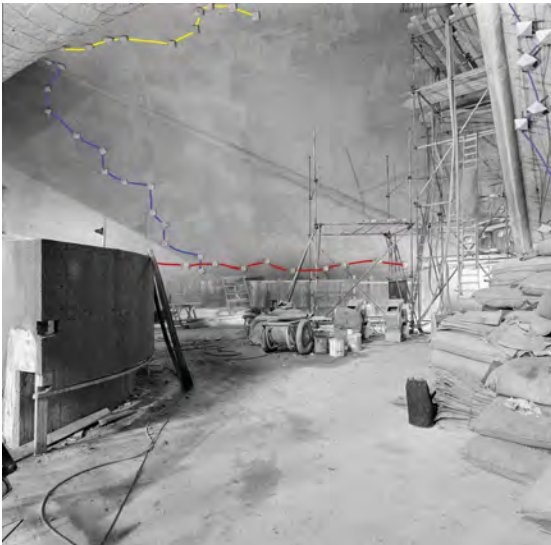
Fig. 2.85: A view in the same direction but further to the right: sound route I (horizontal), in red; sound route II (from route I→A), in blue; route III (B→E→A), in yellow; and route VII (B→U), in purple. Photo by Hans de Boer; colors added by the author, see diagram (fig. 2.76) on foldout on page 154.
