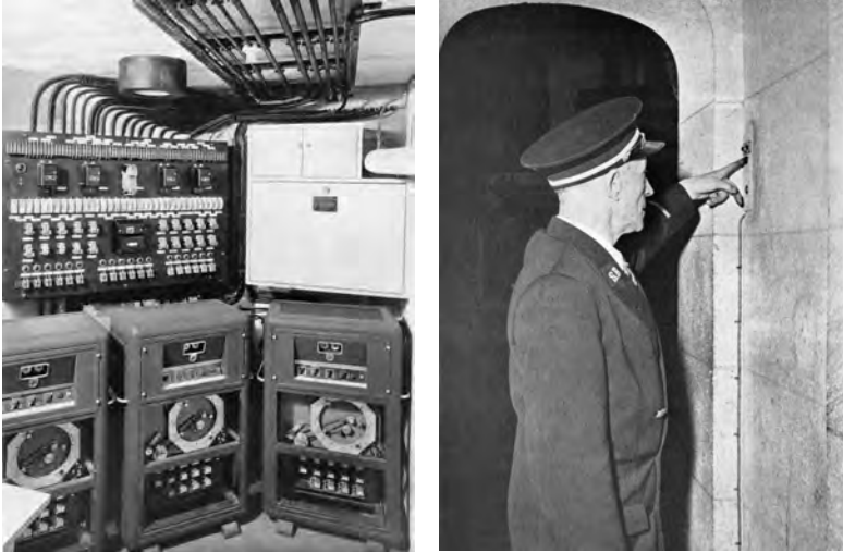
Fig. 2.26 and 2.27: Installation for automated playback of explanatory texts and light switching at the Palais Bénédicte, Fécamp, France (left); a museum guide giving a cue to the machine from one of the exhibition rooms.
