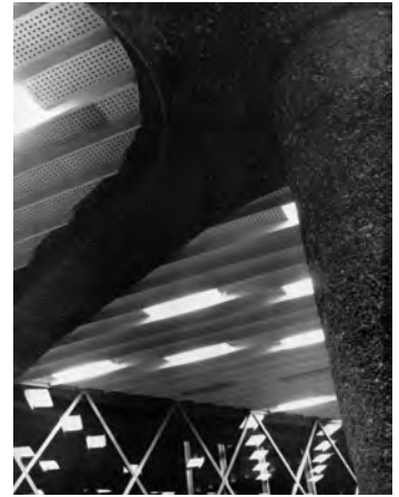
Fig. 2.7: Ceiling with combined distribution of light and sound by Kalff and Tak, installed at the Bank für Gemeinewirtschaft in Cologne, Germany.
