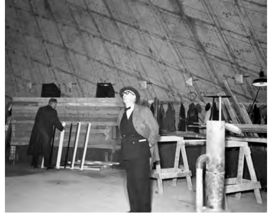
Fig. 2.78: Le Corbusier inspecting the interior of the Philips Pavilion on February 7, 1958. Loudspeakers for the horizontal sound route have been provisionally mounted and covered with plastic to protect them from the impending spraying of the asbestos layer. Their spacing would later be changed at Le Corbusier's request.
