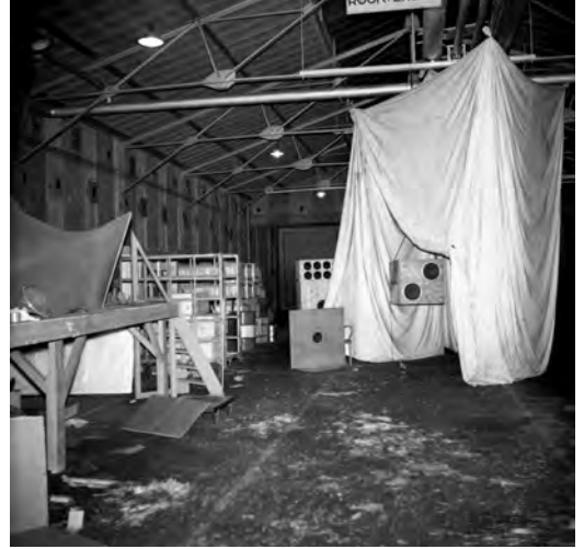
Fig. 2.48 and 2.49: The two full-range loudspeaker cabinets acting as “antiphonal sources” in the front and rear of the garage at Strijp III and loudspeakers for a sound route on the wall. Photos by Anton Buczynski.
