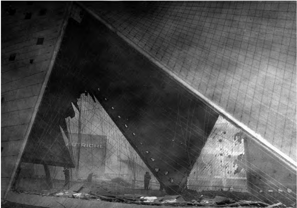
Fig. 2.112: Partially demolished Philips Pavilion, January 30, 1959.
