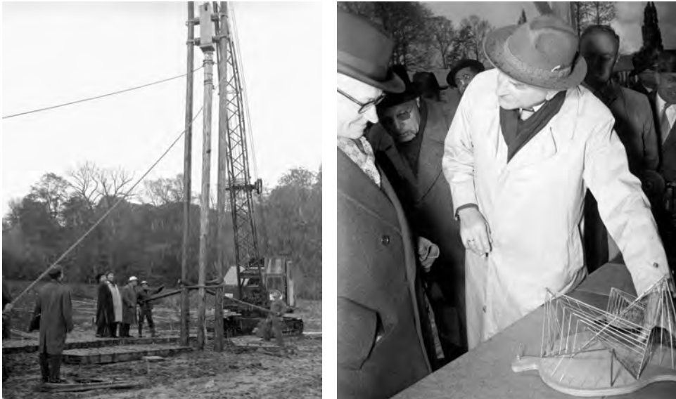
Fig. 2.28 and 2.29: Brussels, May 6, 1957. The first pile for the Philips Pavilion being driven into the ground during a hailstorm (left); Kalff showing a scale model to Charles Spaens, Philips Belgium's deputy manager.
