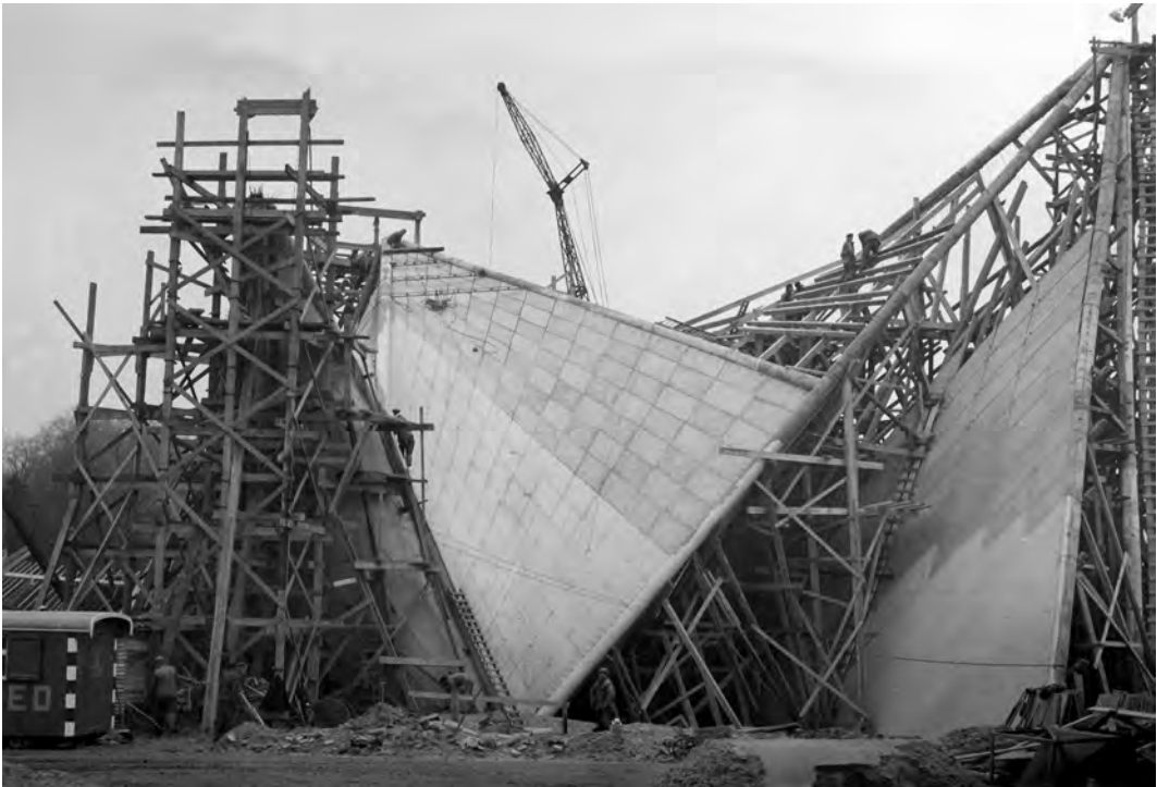
Fig. 2.52: Construction of the Philips Pavilion, August 28, 1957.
