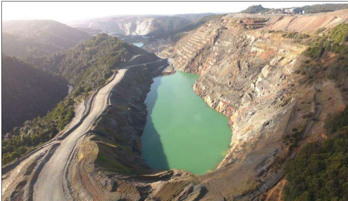
Figure 26: Centre Pit (former CPS) showing water that will be pumped to South Lens
