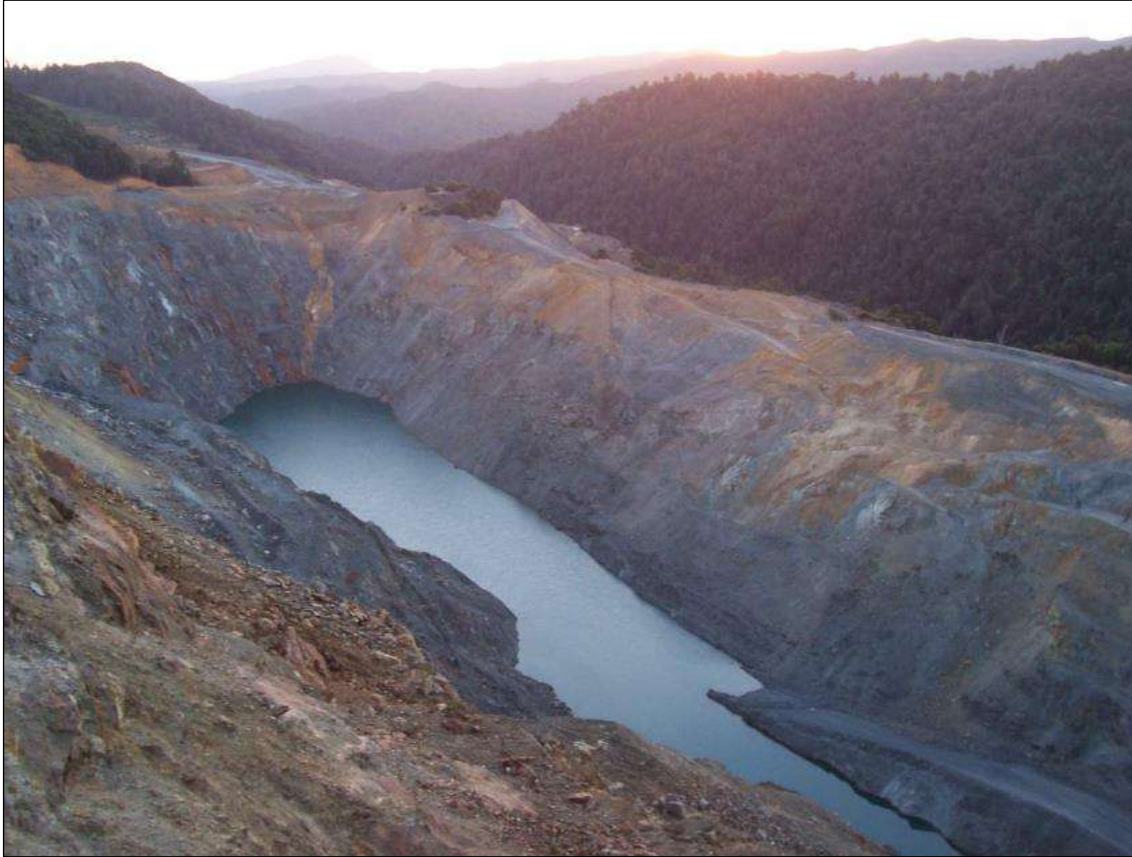
Figure 4: View south across CPS in 2007 after the most recent stage of mining at that location
