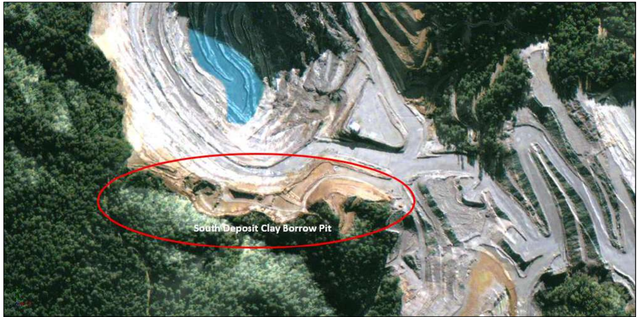
Figure 65: Clay borrow pit location
