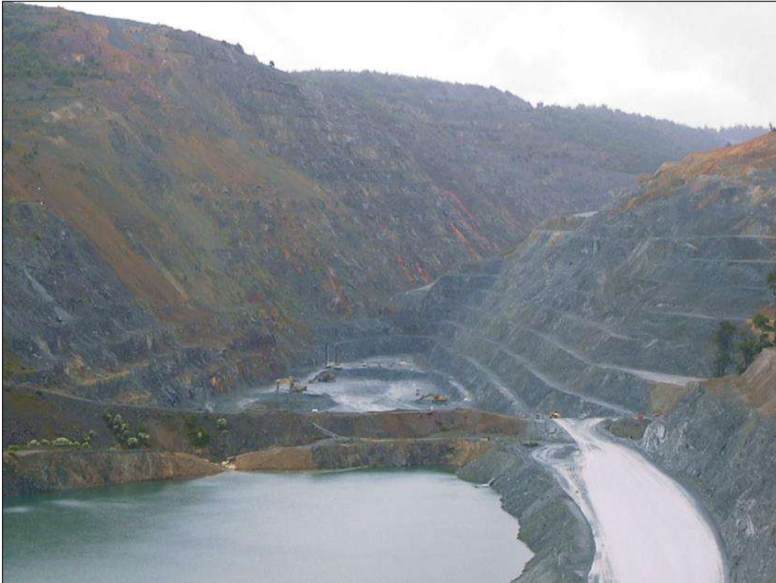
Figure 3: Looking south across South Lens to CPN in 2000 – approximately one year before production ceased
