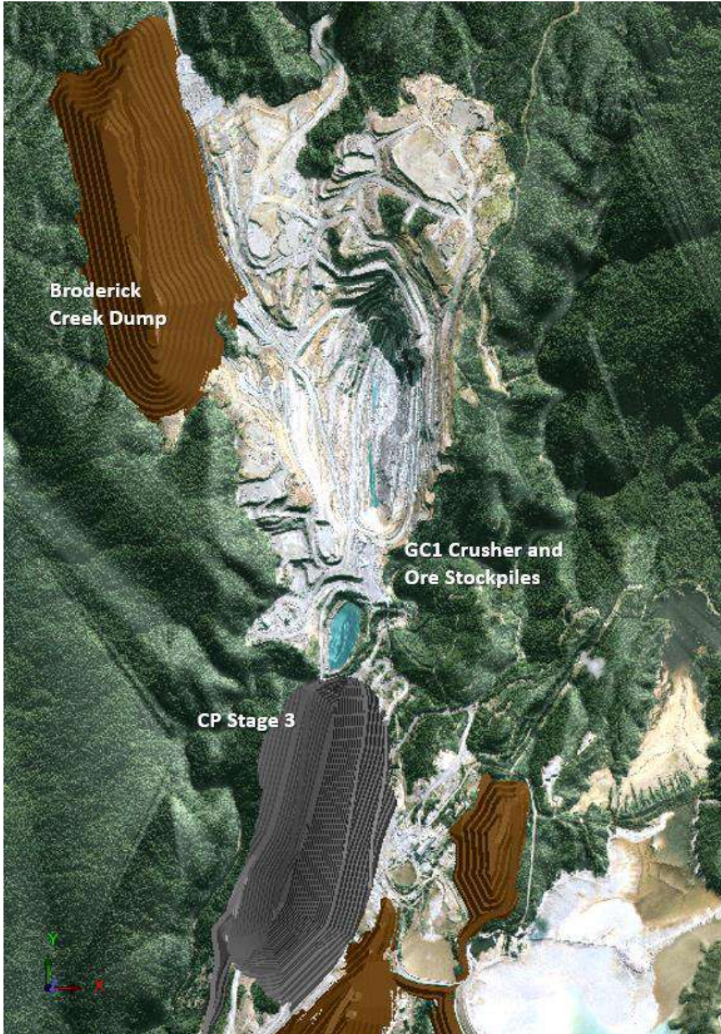
Figure 25: Completed CP Stage 3 and dumps
