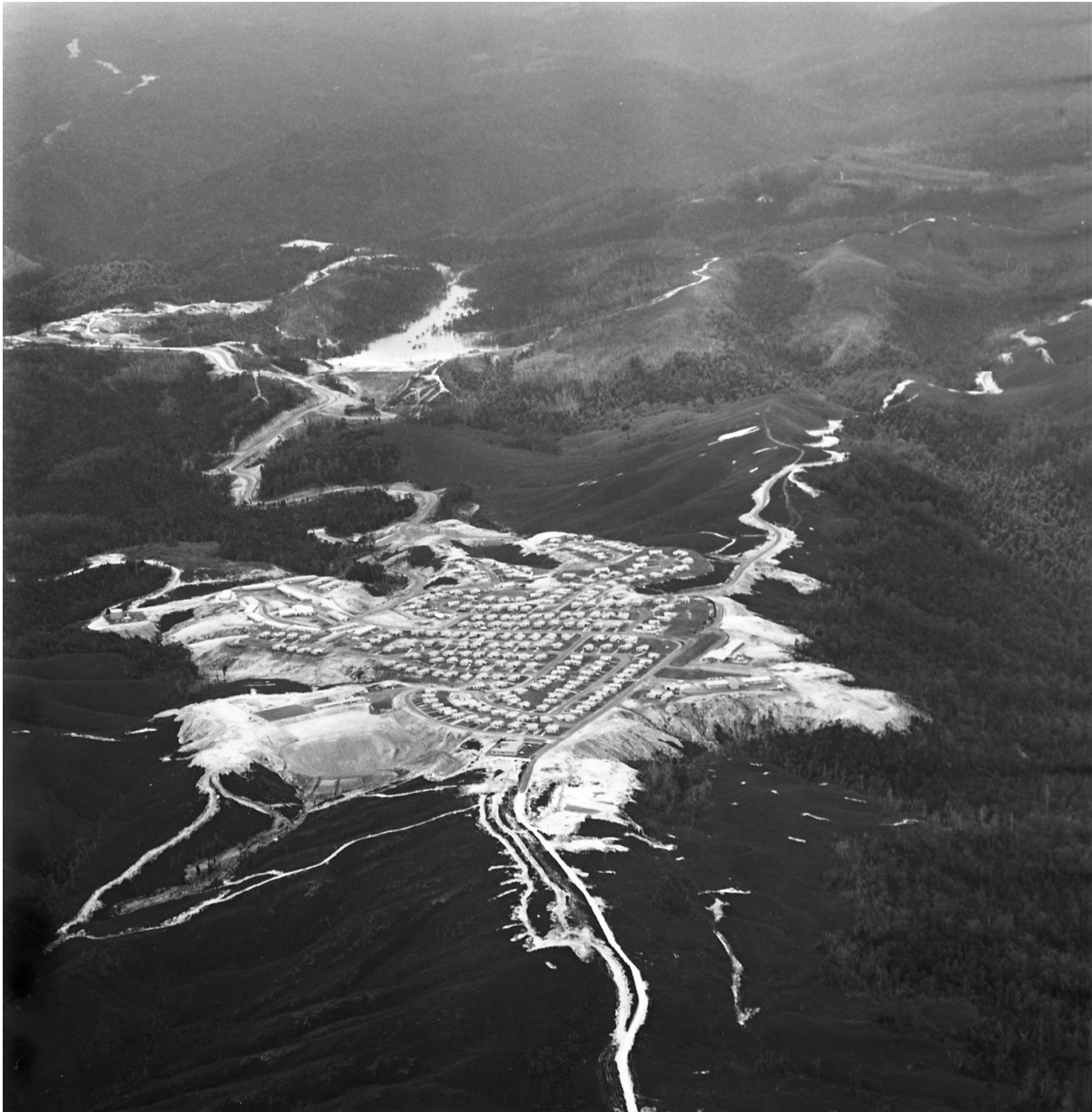
Figure 12: c.1960s photograph of the Savage River township, looking north to the tailings dam and mine site in the distance (TAHO, AB713/1/11918A Photograph - Savage River mine, aerial view, Reproduced with permission).
