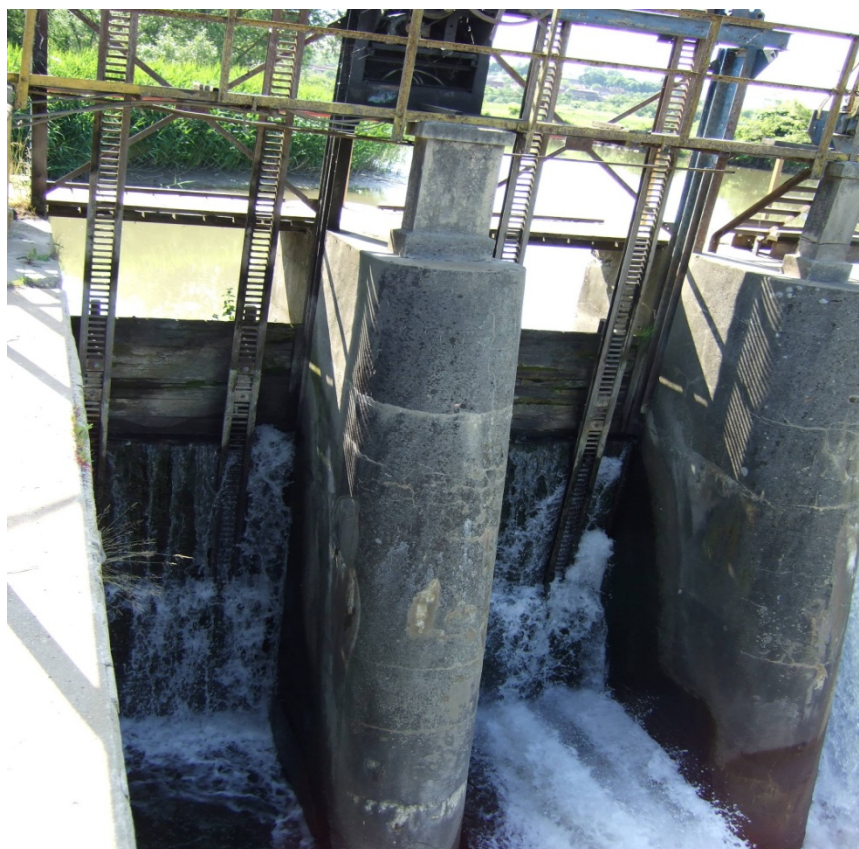
Figure 8: Downstream Mănăstirea Dam.
