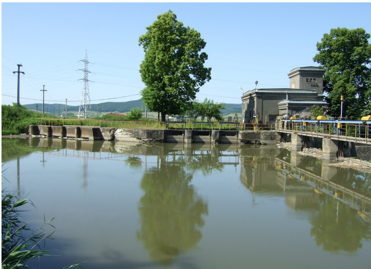
Figure 7: Downstream discharge sill.
