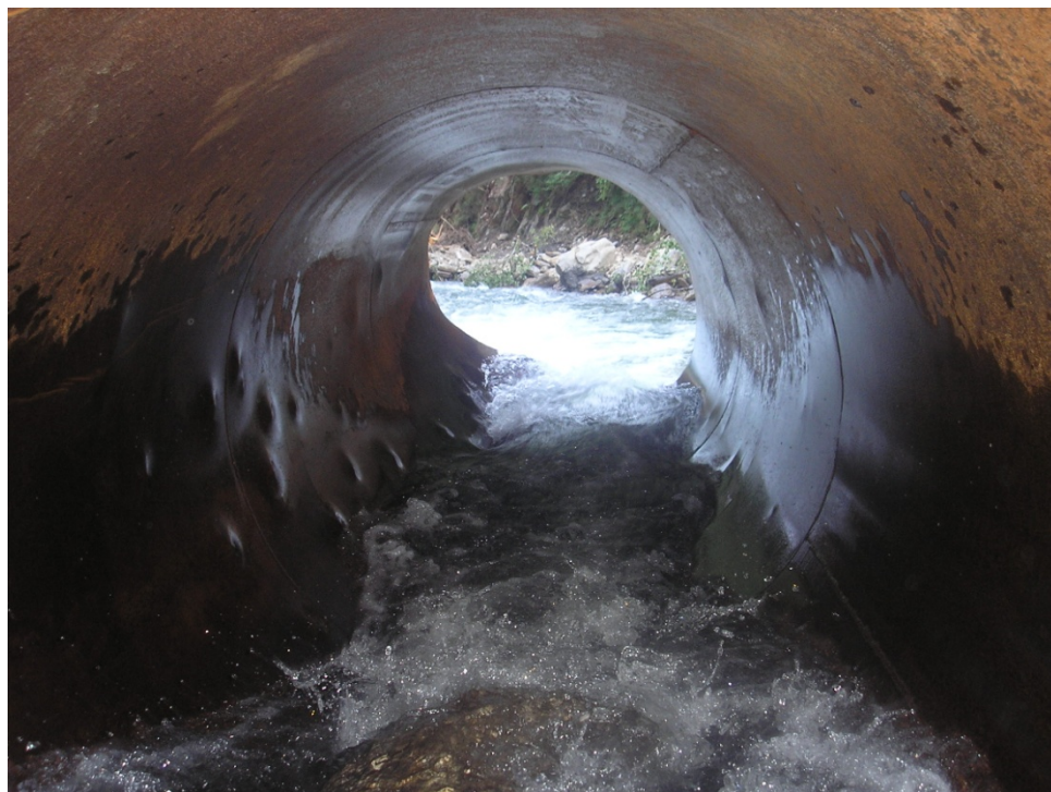
Figure 24: Pipe used for the local hidrotechnical works.
