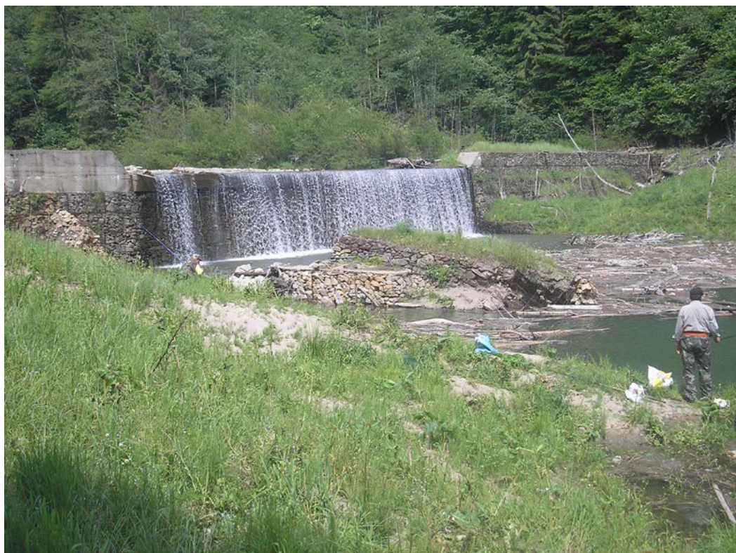
Figure 32: Sampling station 17 on Capra Stream, view from downstream of the concrete anti-bottom sediments dam on the Capra River course at the edge of Vidraru Lake.
