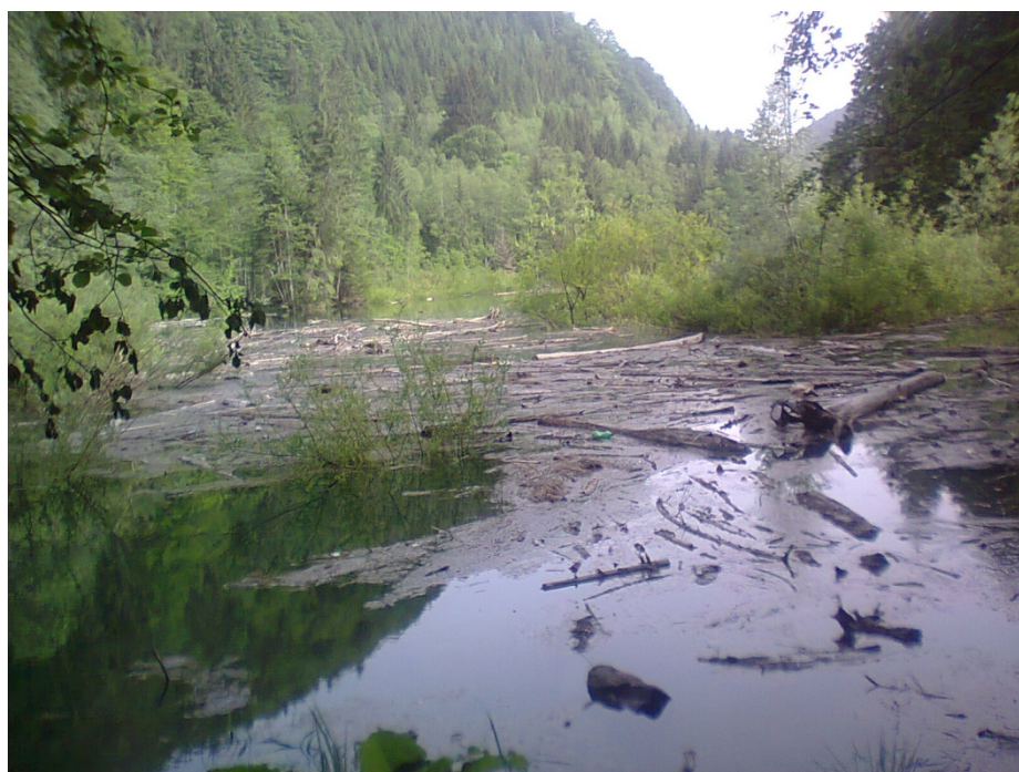
Figure 31: Logs and sediments blocks the dam near the Vidraru Lake during high flows period in S17.
