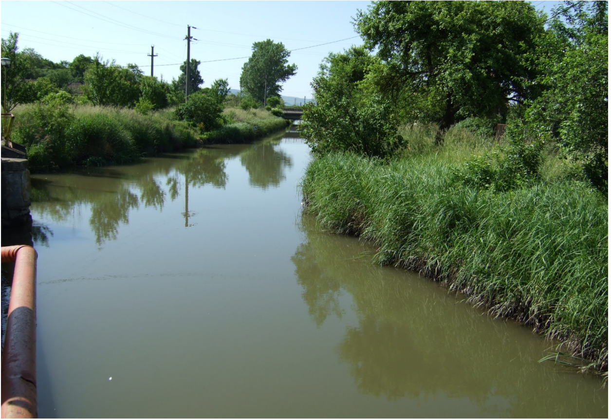
Figure 5: Old outlet small hydropower – upstream (photo: Sofronie C.).
