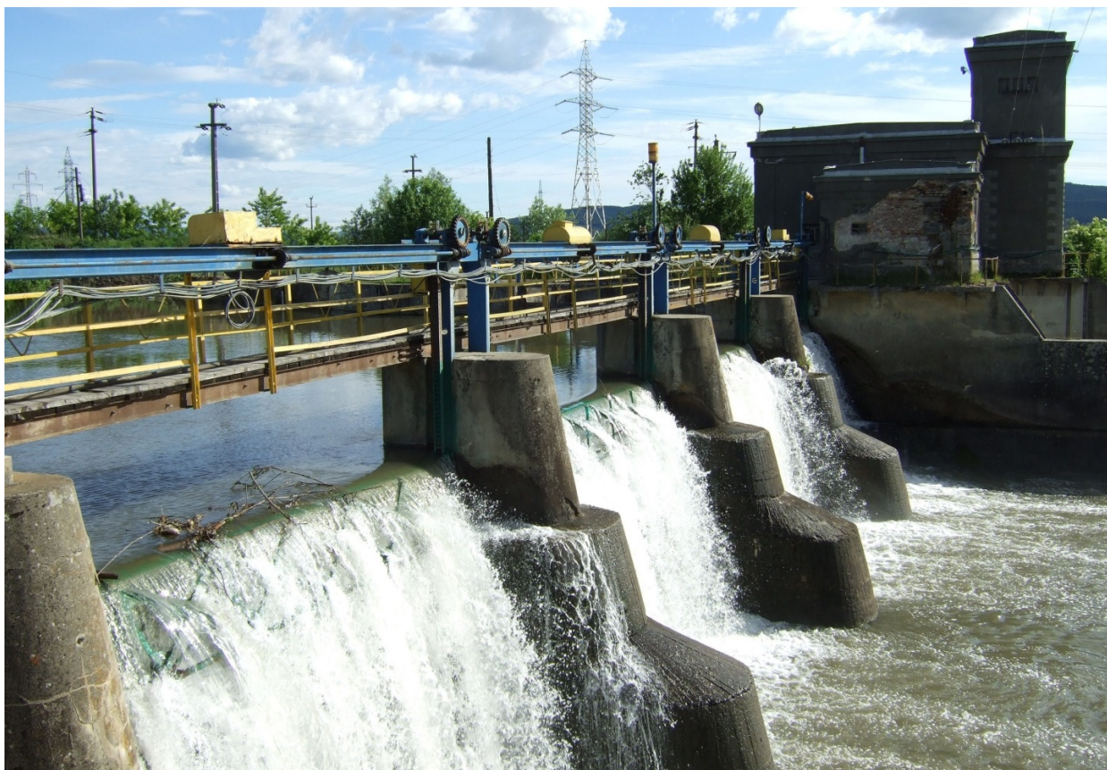
Figure 11: Downstream Mănăstirea Dam.
