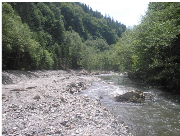
Figure 20: Station 11, buried pipes on bank and riverbed surface diminished with 50%.
