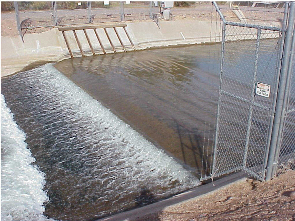
Figure 15c: Electric fields generator for blocking or redirecting the fish positioned before a discharge sill ( http://www.smith-root.com/ ).
