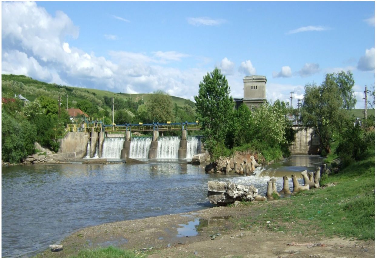
Figure 10: Downstream Mănăstirea Dam.
