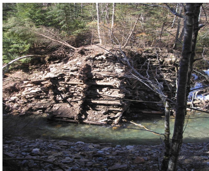
Figure 21: Near the station 11, remains of old rocks and logs dam used for lodgs rafting.
