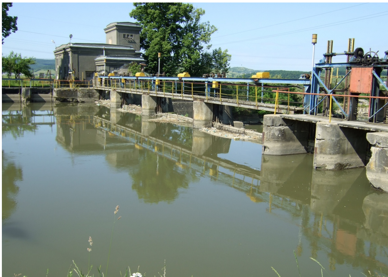
Figure 3: Dam – upstream view (photo: Sofronie C.).
