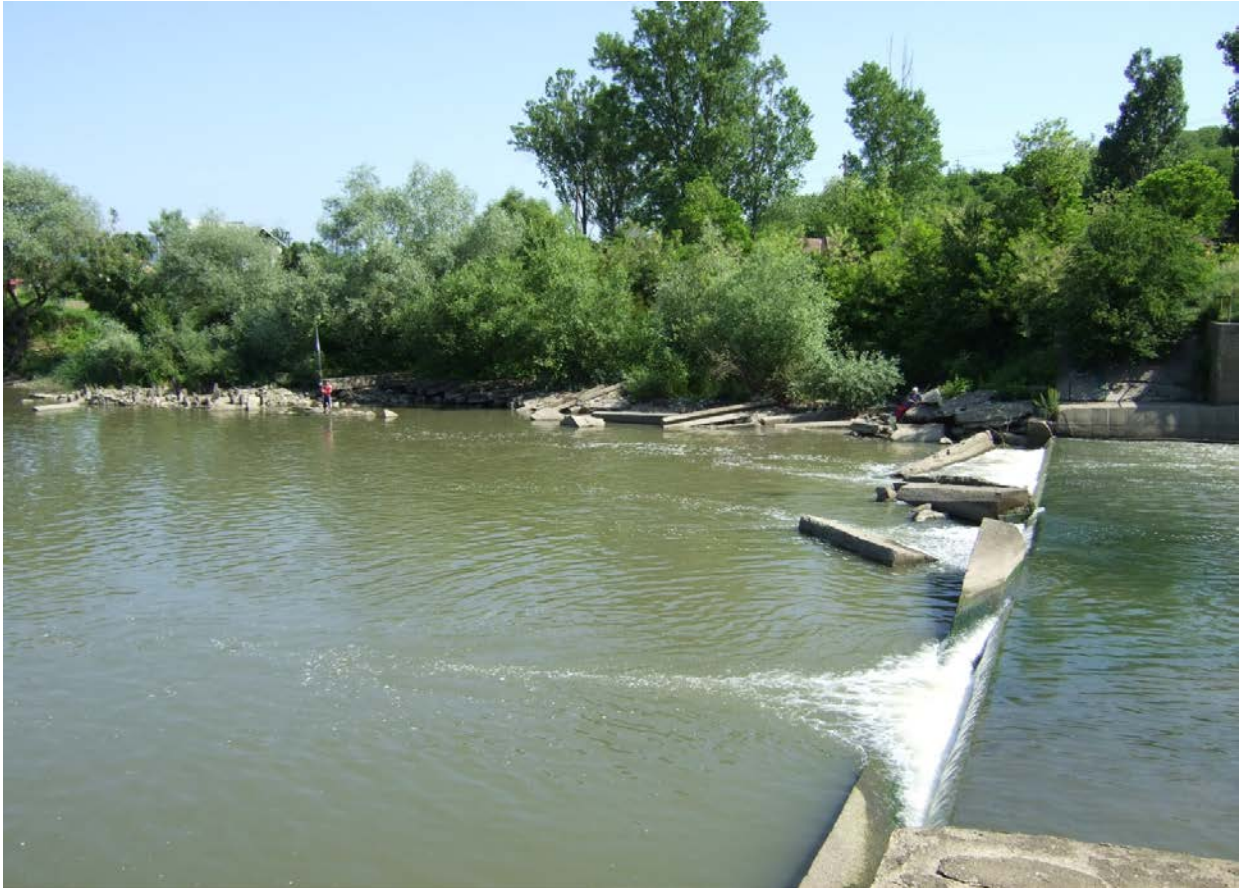
Figure 9: Downstream discharge sill.
