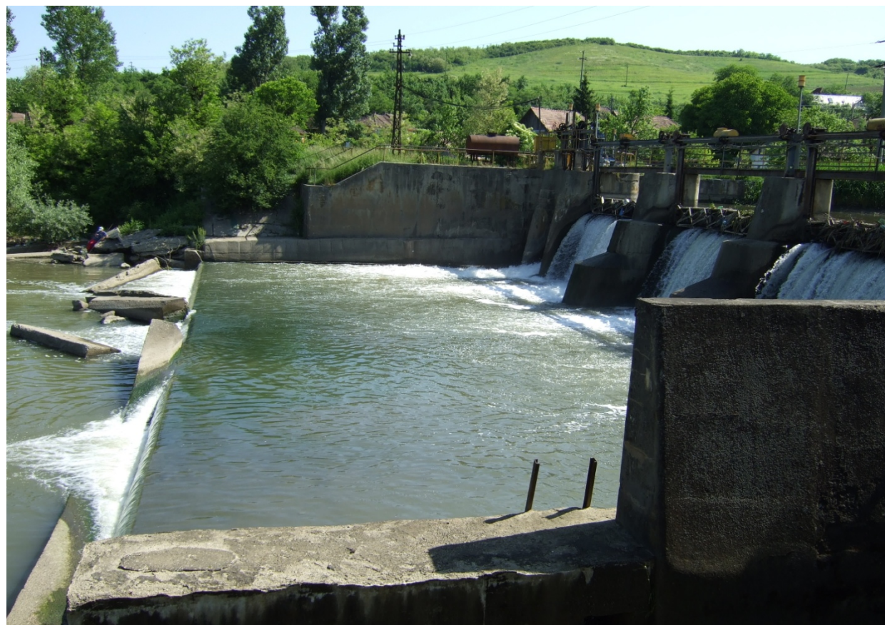
Figure 4: Dam – downstream view and toe basin (photo: Sofronie C.).
