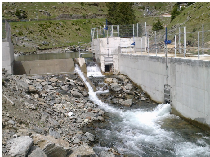
Figure 9: Capra Stream – micro hydropower plant Capra I.
