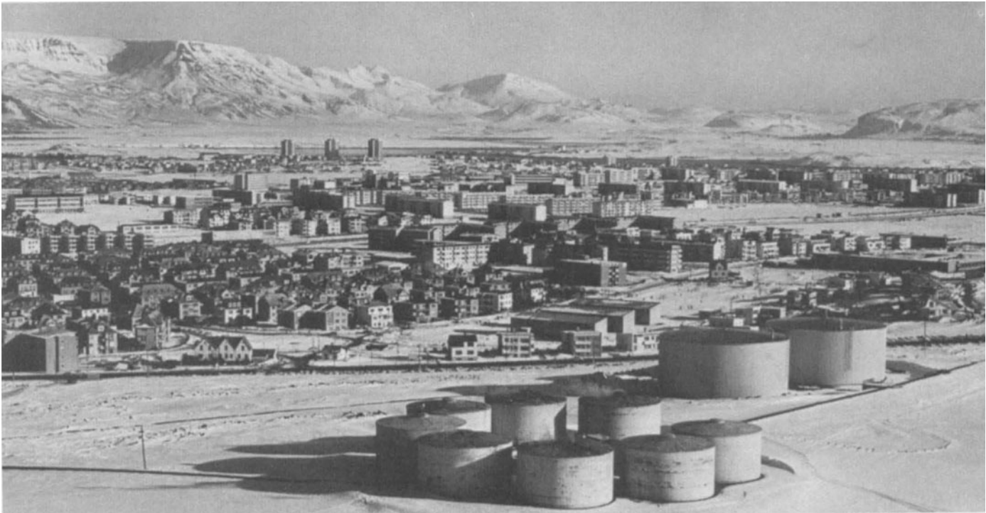
Fig. 9. Hot water reservoirs serving the Reykjavik geothermal heating system. (Photo by Mats Wibe Lund.)
