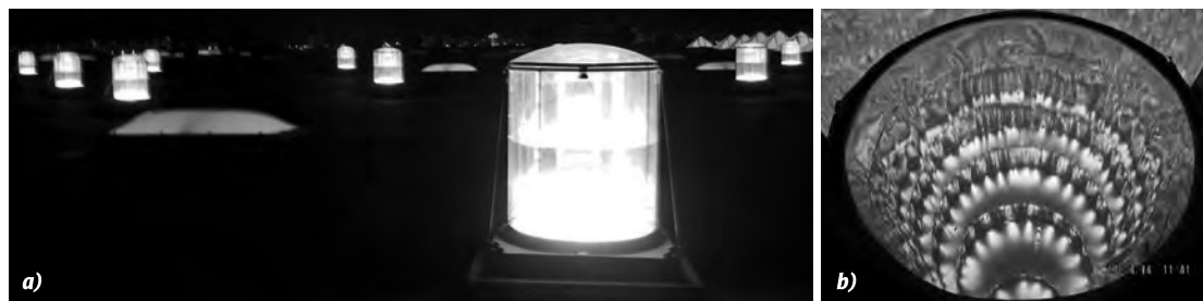
Fig.1. The illumination manifold as a result of “selling” reflections of the LED module luminous flux (a) and mirror reflection LED module (top view through a manifold in the channel of hollow tubular light guide) (b)
