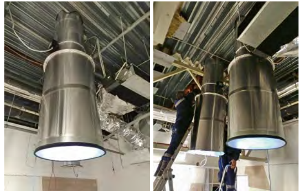
Fig.7. HLC “Solar LED-S” in the “Meeting room “ (installation process). ALB is located in the space of the technical floor, located above the ceiling of the “Meeting room” under the roof (internal design)
