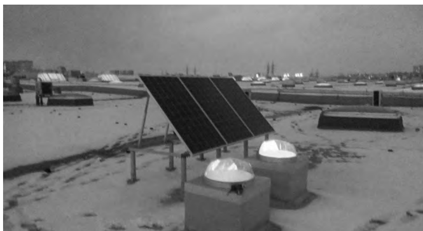
Fig.9. View on the roof: HLC- inlet and solar panels
