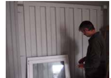
Mark measures up the salvaged window that will be fitted into the back wall of this container.
