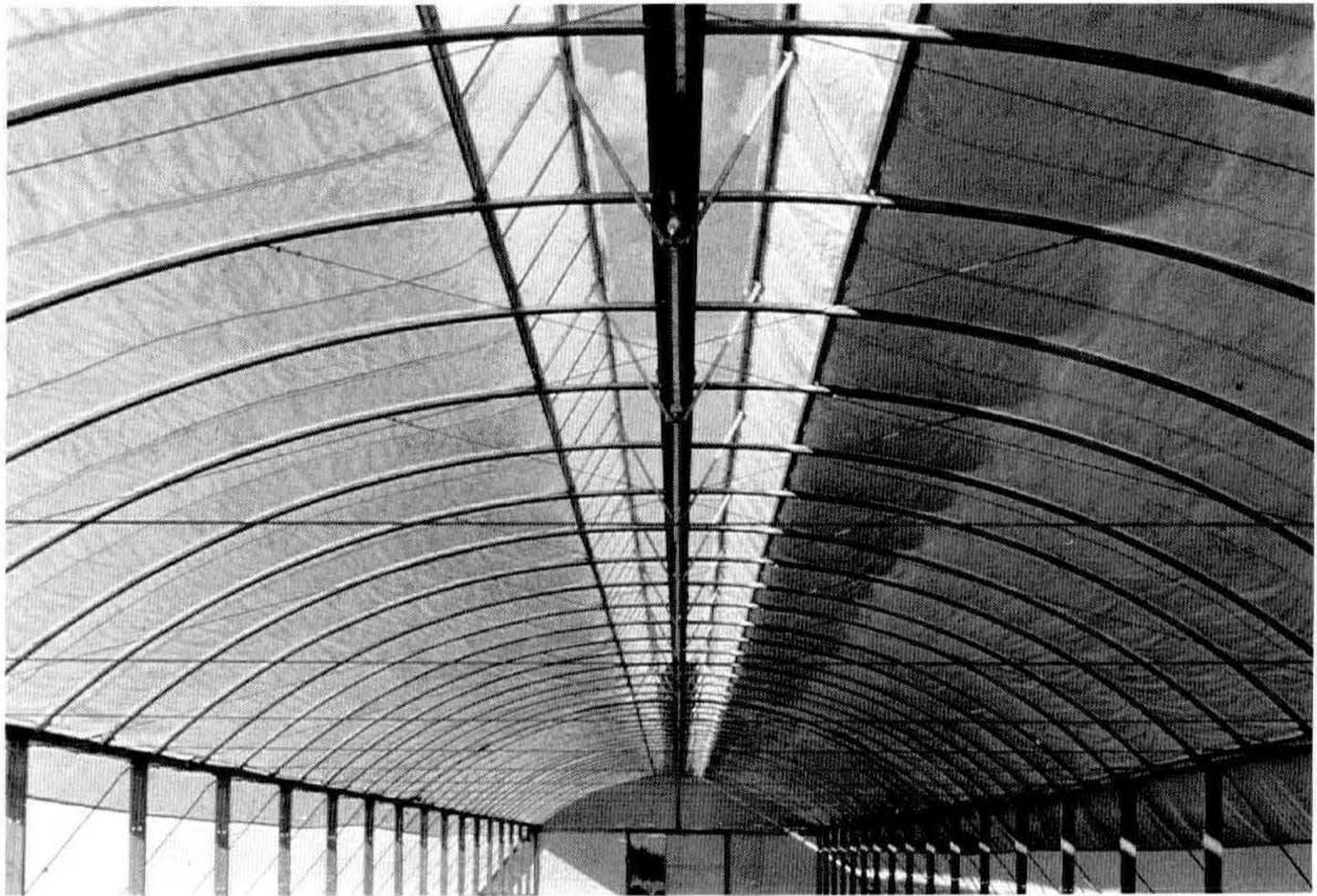
Figure 2. Roof-vented poly-covered quonset structure.
