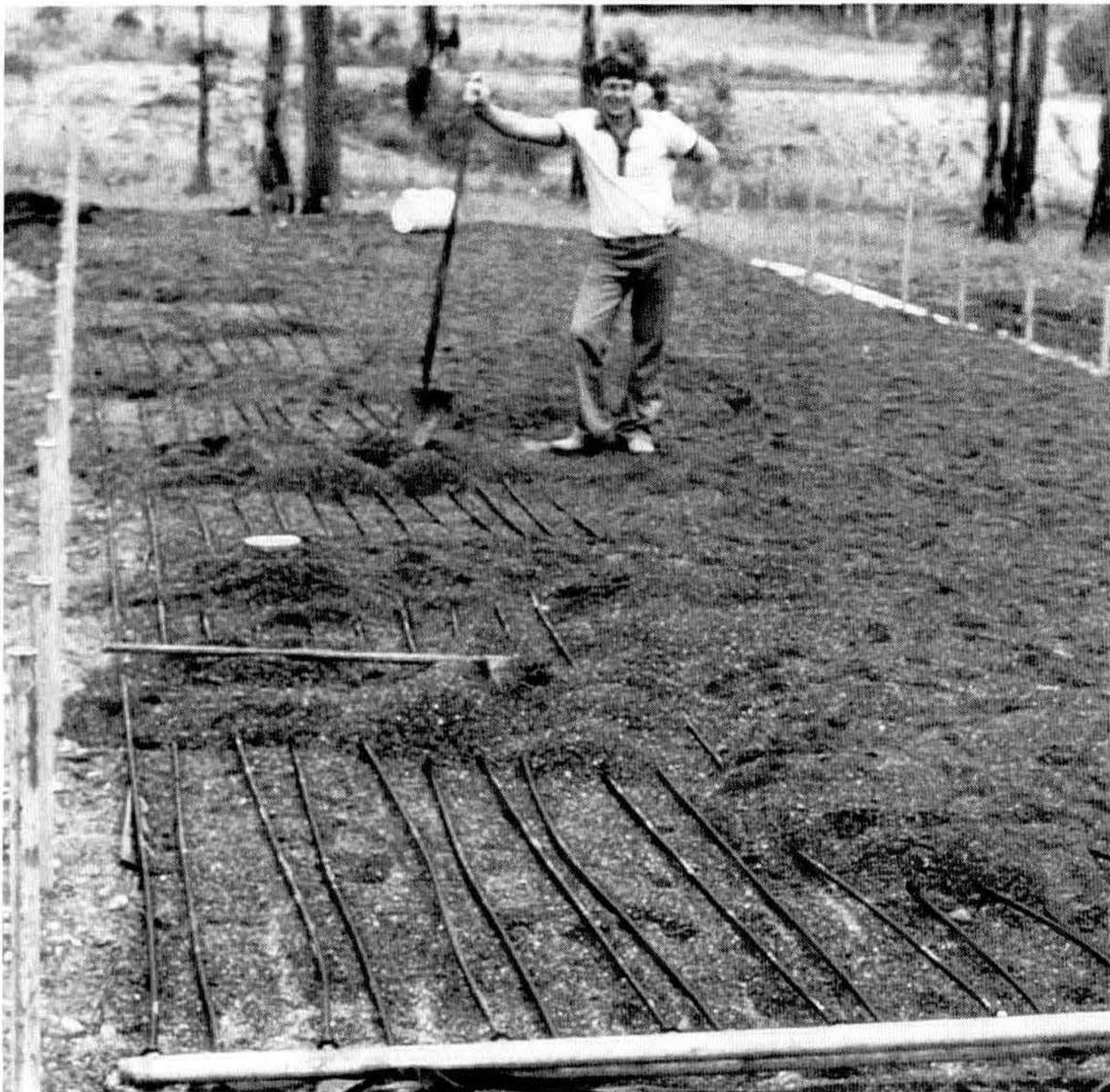
Figure 4. Heat lines are laid in a sand bed then covered with matting.
