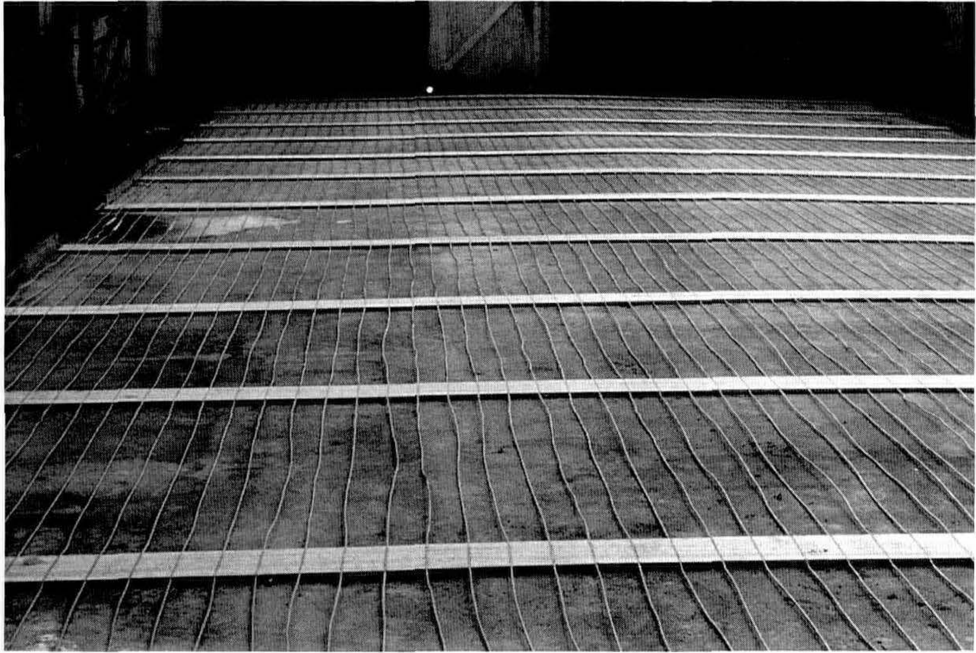
Figure 3. Bottom heat in the floor.
