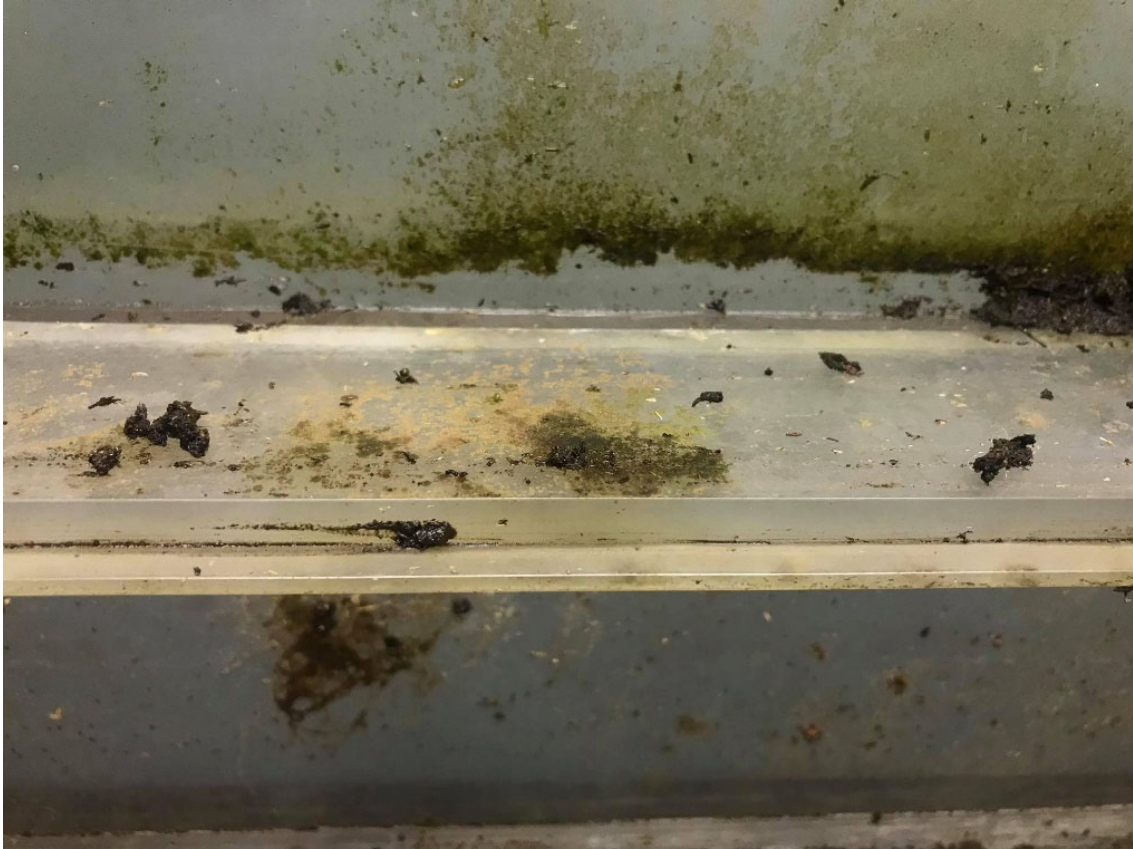
There is a grooved lip that holds the grating in place.
