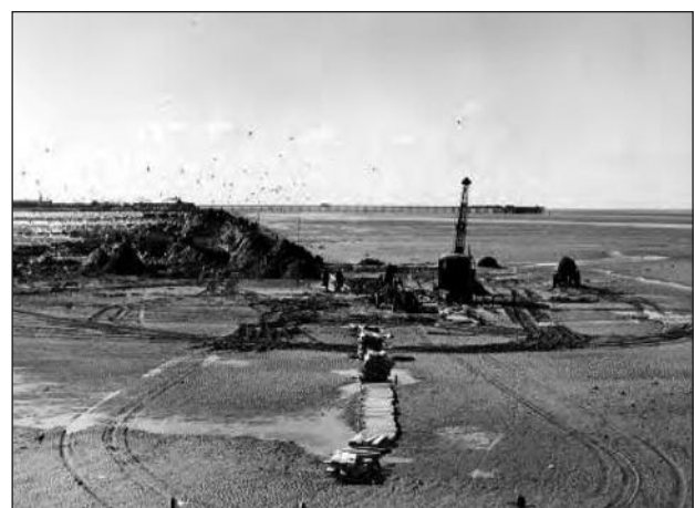
Plate 3. Construction of Marine Drive, looking south east, estimated mid 1960s. The black dots above the construction site are large numbers of seagulls in the picture due to the road being backfilled with household waste. (Image held in SMBC archive).
