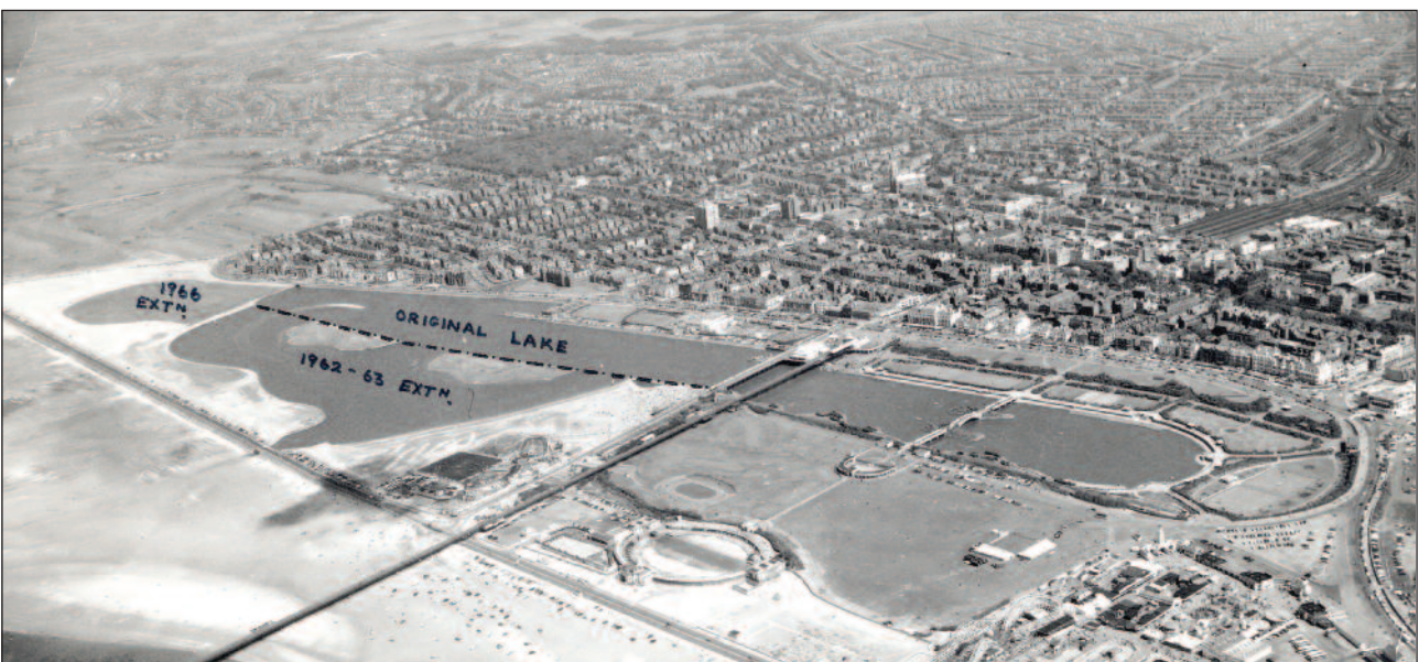
Plate 5. Photograph of Marine Lake, looking west, showing dates of construction, c.1966. (Image courtesy of SMBC).
