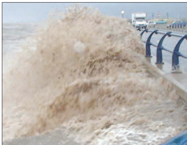
Plate 8. Wave overtopping at the sluice gates, Marine Drive, 2005. (Image courtesy of Terry Hedges).
