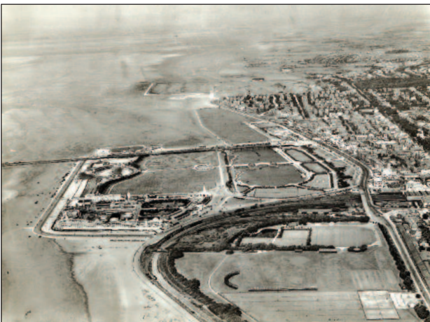
Plate 4. Aerial photograph of Southport foreshore looking north west, pre construction of the Coast Road and reclamation to create the Marine Lake extension, estimated mid 1950s. (Image courtesy of SMBC).
