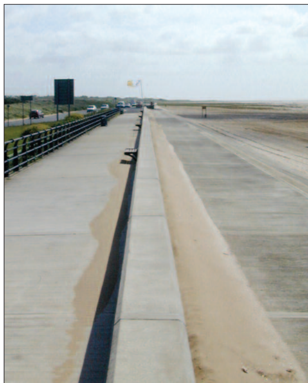
Plate 11. Accumulating wind blown sand on the sea wall. (Image held in SMBC archive).
