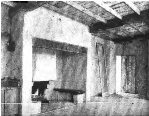
'Fireplace has cosy ingle seats of hewn bush timber.' (Source: Johnston, 'Built from the good earth', AHB, June 1948, p29)
