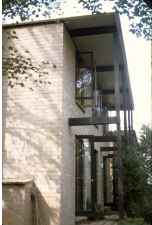
Rear elevation of the Swift's two-storey block – deck since expanded a new timber deck has been constructed (Source: Peter Wille, SLV, H91/244/1567)
