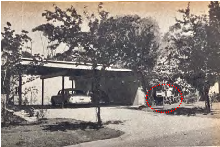
Photograph of carport and façade of Beddison/Swift House from Crown Road Note horizontal timber post box, which is extant, circled (Source: 'Two Families Share View', AHB , April 1965, p23)
