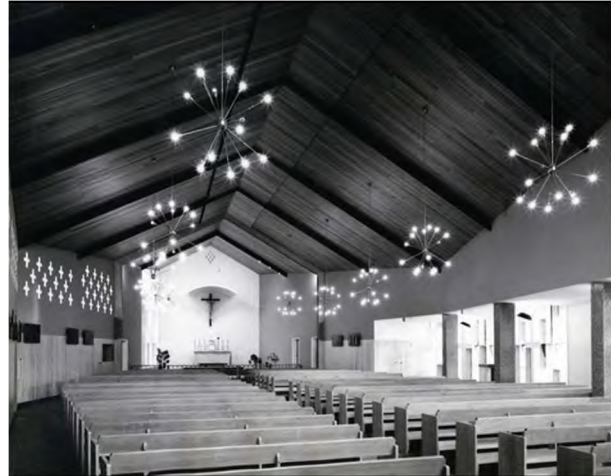
Original nave showing 'starburst' light fittings (replaced) and steel beams (Source: www.ivanhoecatholics.com/parishhistory.htm )
