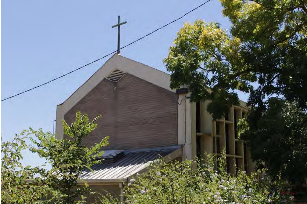
South (rear) elevation with later addition skillion volume in the foreground and section of window wall with 'random' muntin bars on right of frame
