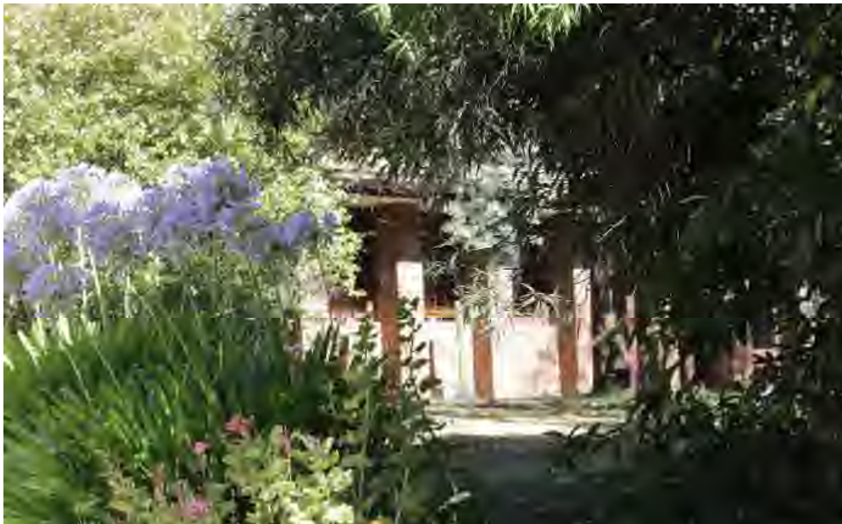
Landscaped filtered view to west wing from street, note different bay treatment with casement windows/ low brick wall (left) and floor-to-ceiling windows (right)
