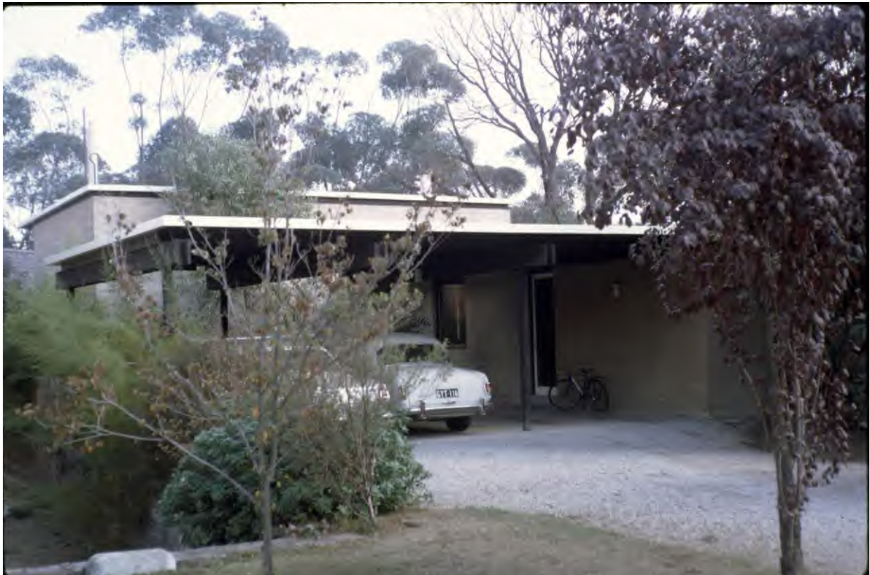
Beddison/Swift House from Crown Road (Source: Peter Wille, SLV, H91/244/1569)
