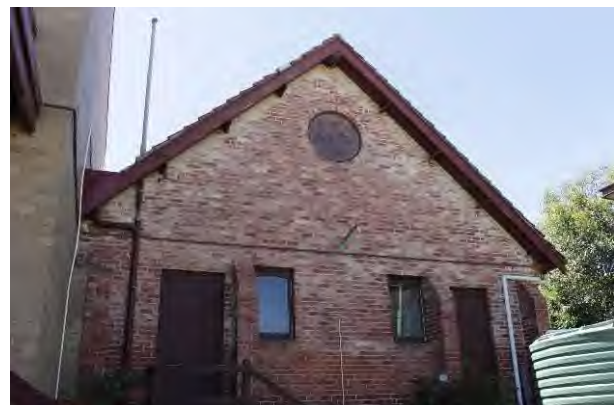
Earlier Hall – west elevation
