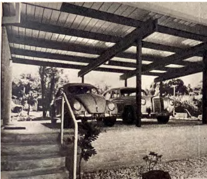
Photograph of internal front courtyard to carport ceiling (Source: 'Two Families Share View', AHB , April 1965, p23)
