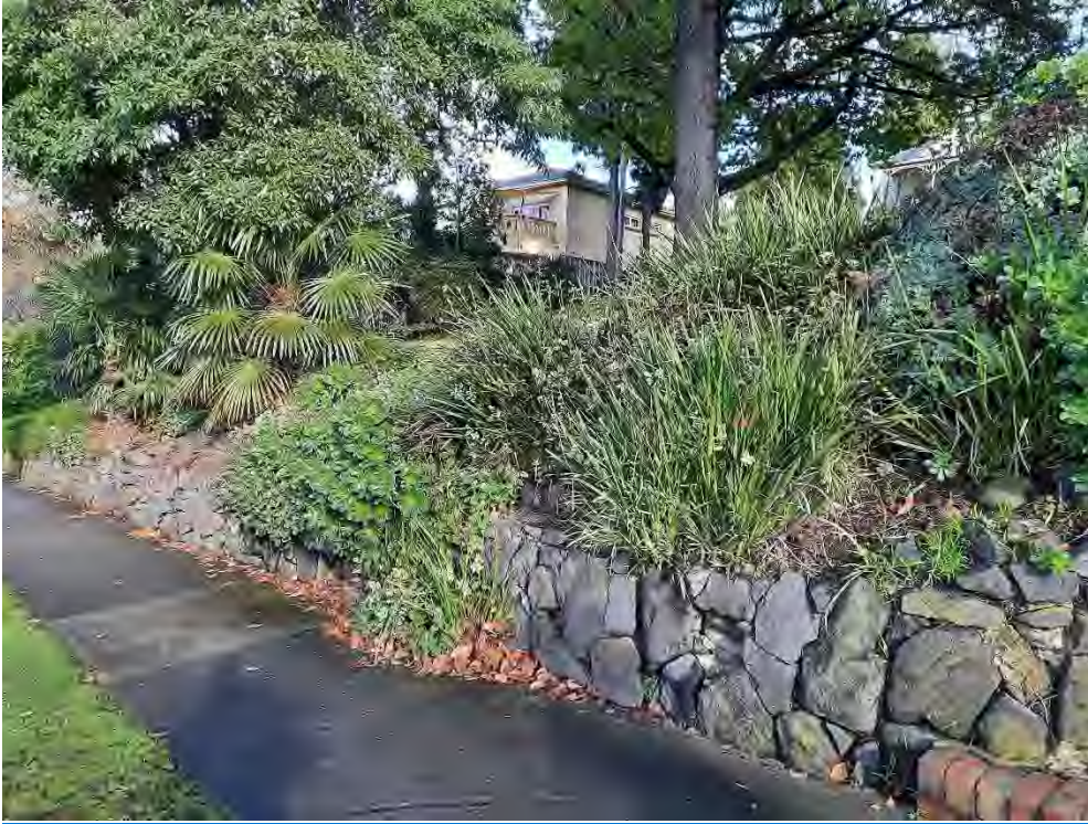
The drystone retaining wall to the front boundary dates to the North period of ownership (circa mid-20 th century)
