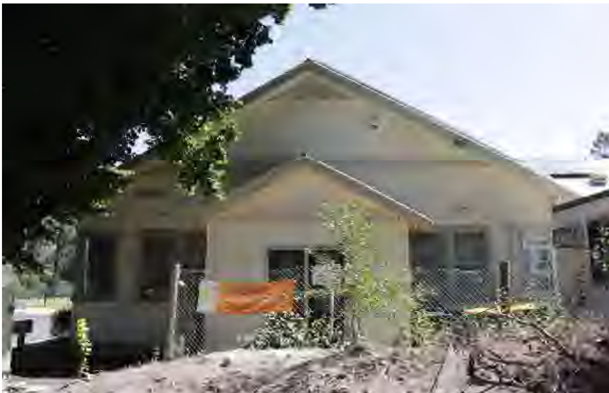
1925 façade – note distinctive fenestration and retention of signage panel
