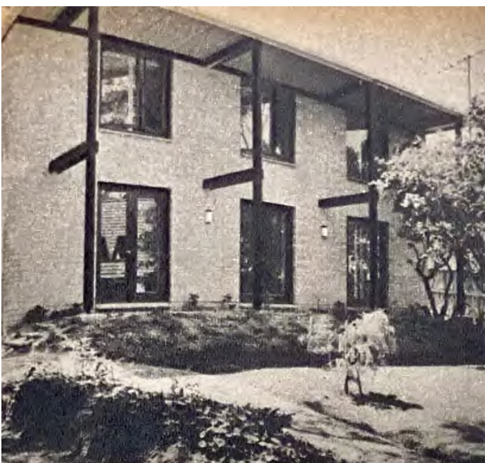
Original R ear frontage of the two-storey unit from back yard (Source: 'Two Families Share View', AHB , April 1965, p23)
