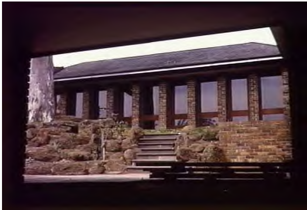
Eastern wing from carport (Source: Peter Wille, SLV, H91.244/1702)
