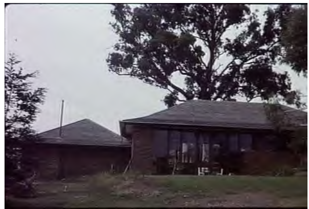
Rear elevation carport (note initially solid wall) and central wing (Source: Peter Wille, SLV, H91.244/1686)
