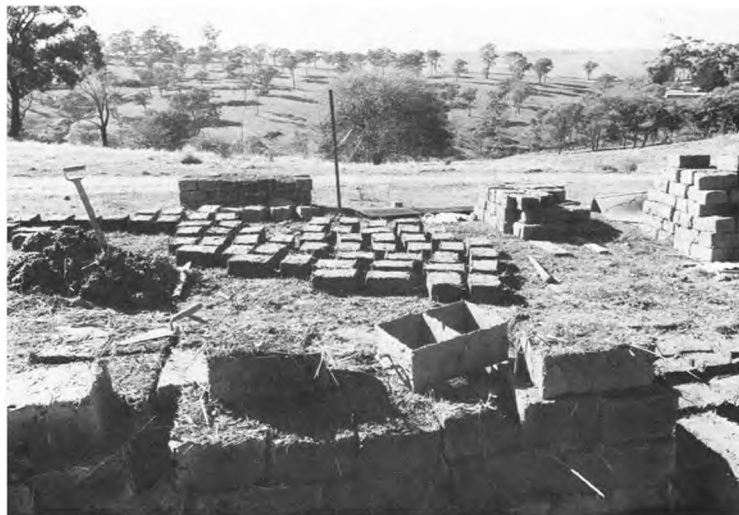
Clay bricks in production, undated, unspecified site (Source: Alistair Knox, Living in the environment , 1978)
