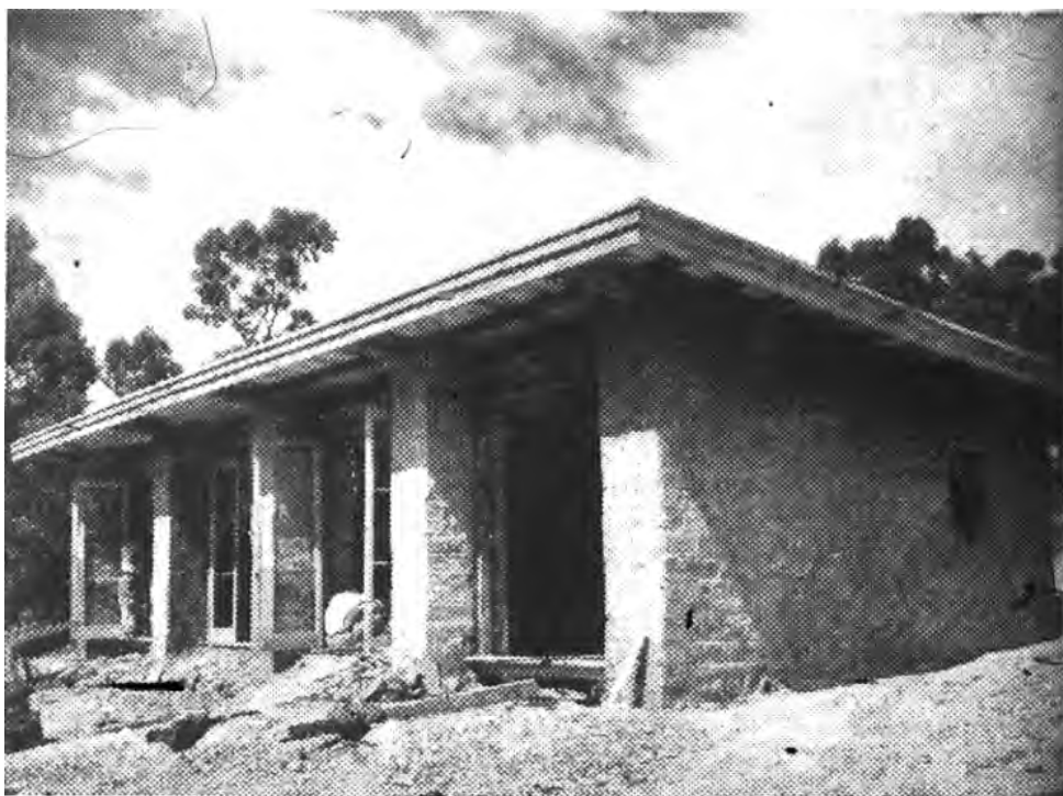
Close-up of the original north (rear) elevation of English House , showing original scale: 'Piers accentuate depth of wall near French windows.' (Source: Johnston, 'Built from the good earth', AHB , June 1948, p29)
