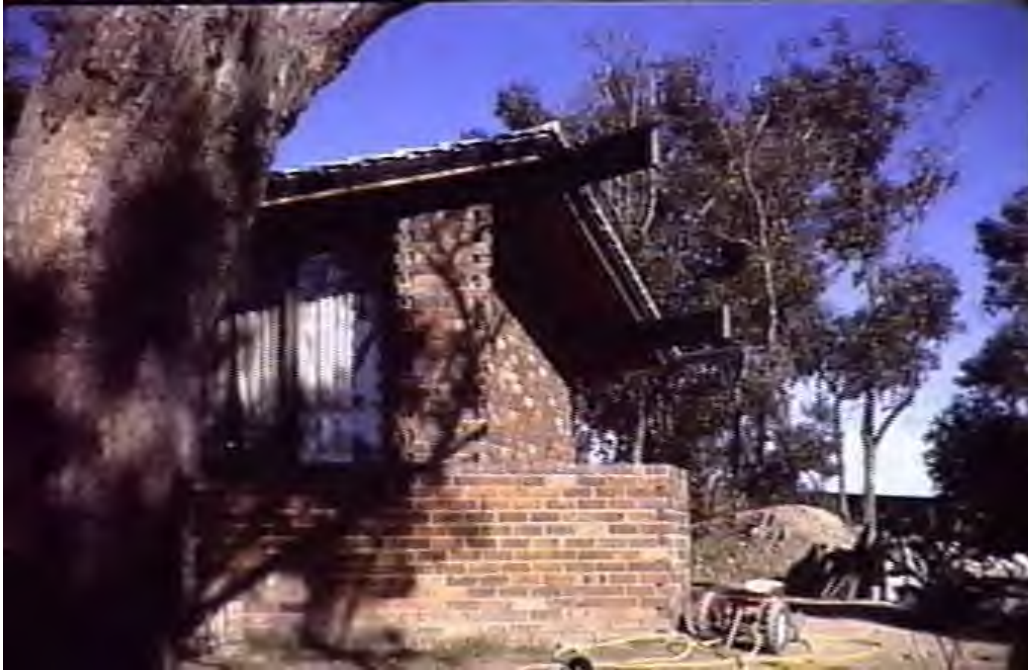
Rear wing (south), during or soon after construction (Source: Peter Wille, SLV, H91.244/1738)
