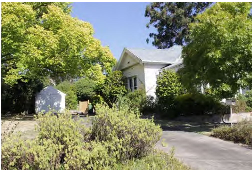
View to rear garage and north elevation with projecting gabled wing
