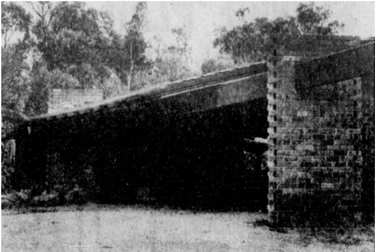
‘Heavy laminated beams supported on brick piers enclose the carport of Charles Duncan’s design at Lower Eltham’ (Source: Barker, “The Age” — RAIA Citation Award No. 34’, Age , 15 May 1972, p11)
