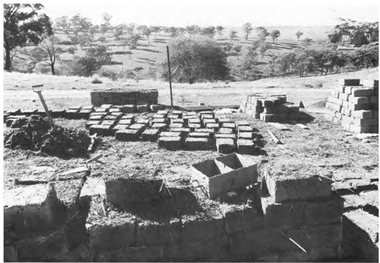
Clay bricks in production, undated, unspecified site (Source: Alistair Knox, Living in the environment , 1978)
