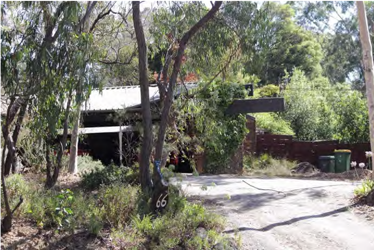
Carport with timber beams prominent
