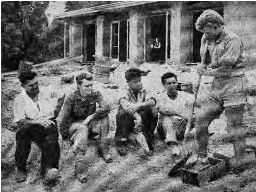
'Gordon Ford stamps mud into a brick mould, while Laurie Mayfield (left), Miss Sonia Skipper, Alistair Knox and Tony Jackson look on.' North (rear) elevation of English House in the background (Source: Johnston, 'Built from the good earth', AHB , June 1948, p28 – courtesy of Miles Lewis, Australian Building: A Cultural Investigation )
