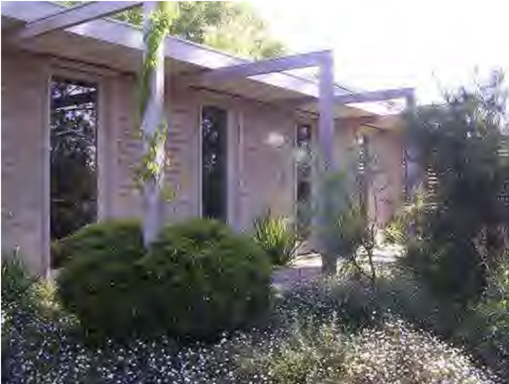
Close-up of north elevation, circa 2005
