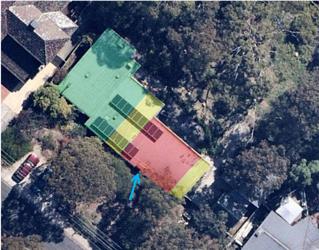
Close-up aerial photograph of English House with approximate extent of construction phases shaded Red shading, 1947 – note the blue arrow indicates the location of the external chimney breast and related internal fireplace and inglenook Yellow shading, mid-1960s additions Green shading, circa 1996 additions (Source: Nearmap, March 2021)
