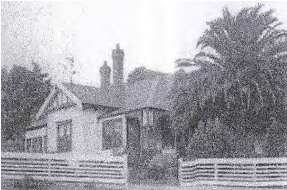
Graceburn , north-west corner, circa 1957 Note two chimneys on north side, since removed, and likely original colour scheme (Source: Heidelberg Historical Society)
