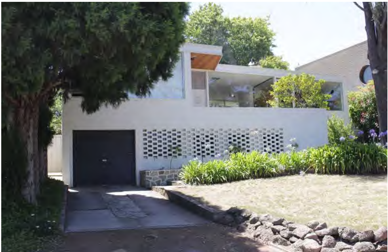
Front, showing extent of concrete paving, and areas of random stone/crazy paving
