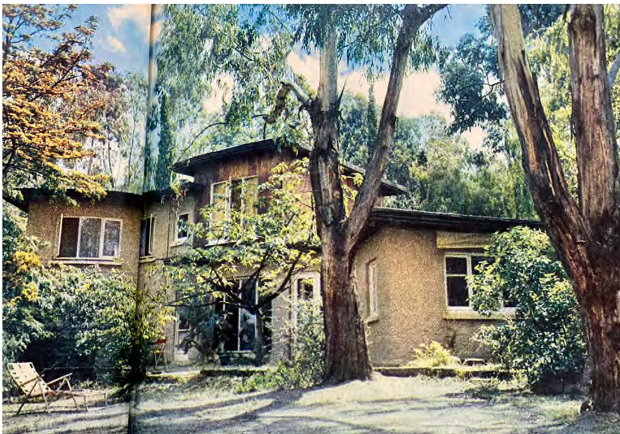
Photograph of the east elevation, note that the page crease obscures the extent of the south wing The north wing (left of frame) was later extended (Source: Bennetts, 'Did The House Live Up To Expectations', AHB , March 1969, pp6-7)
