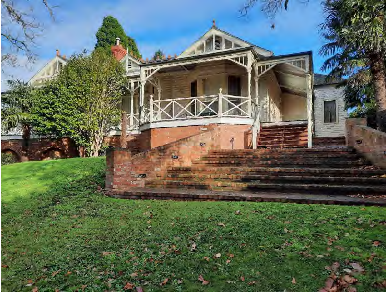
Royd's extant façade, north end showing the forward extension of the verandah, new stair, and the rear additions (behind the northern return of the verandah)
