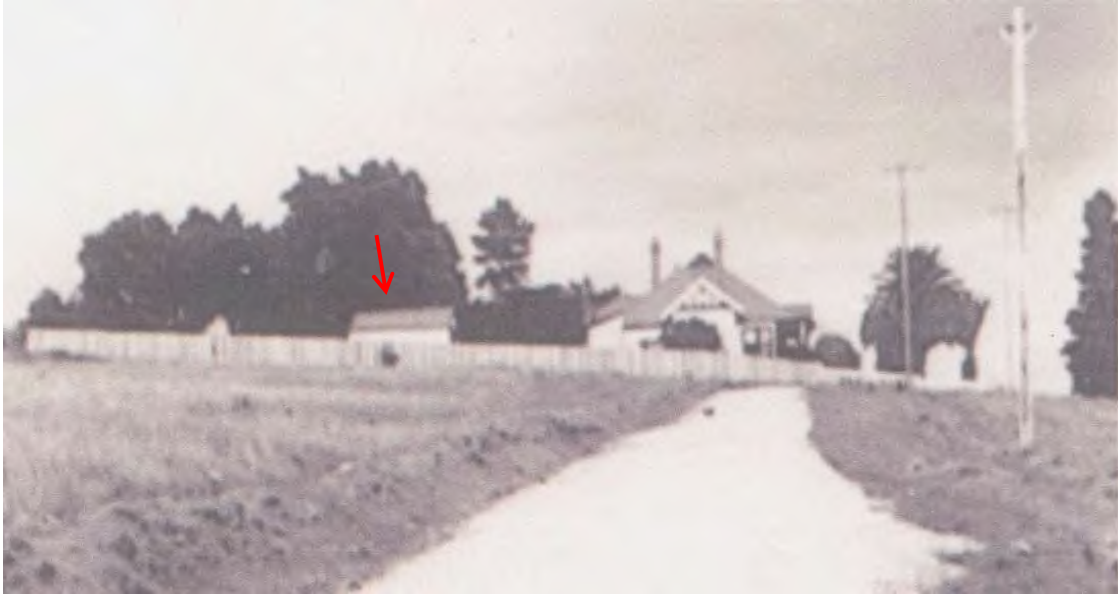
Graceburn , view from the north along Quinn Street, circa 1957 The outbuilding (red arrow) may be the extant timber garage in its original position (Source: courtesy of Heidelberg Historical Society)
