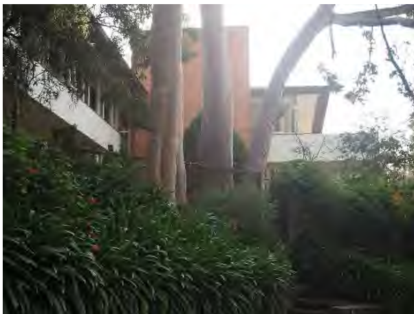
Junction of east and north wings - Streeton Crescent
