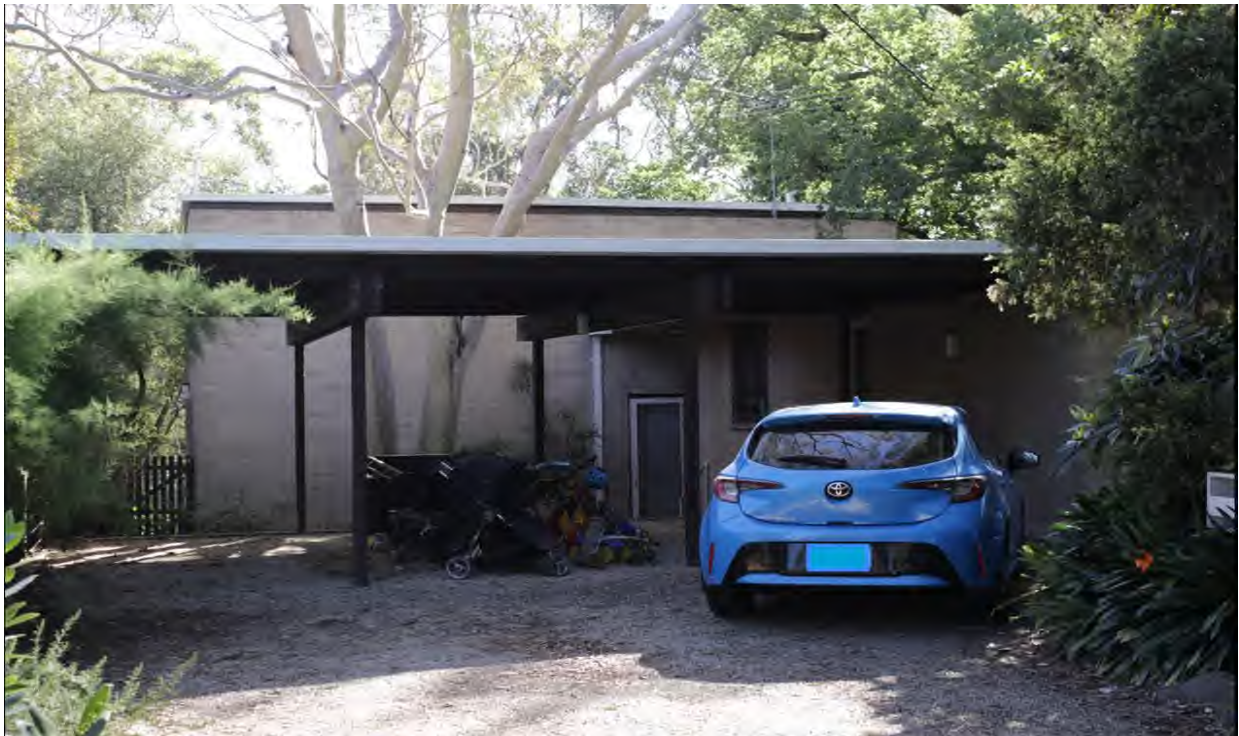
View to carport with the two-storey Swift's block, behind the sunken courtyard, evident to the rear
