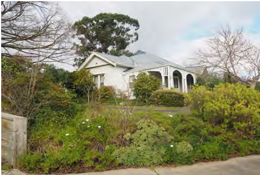
View to north elevation and northwest corner of front verandah
