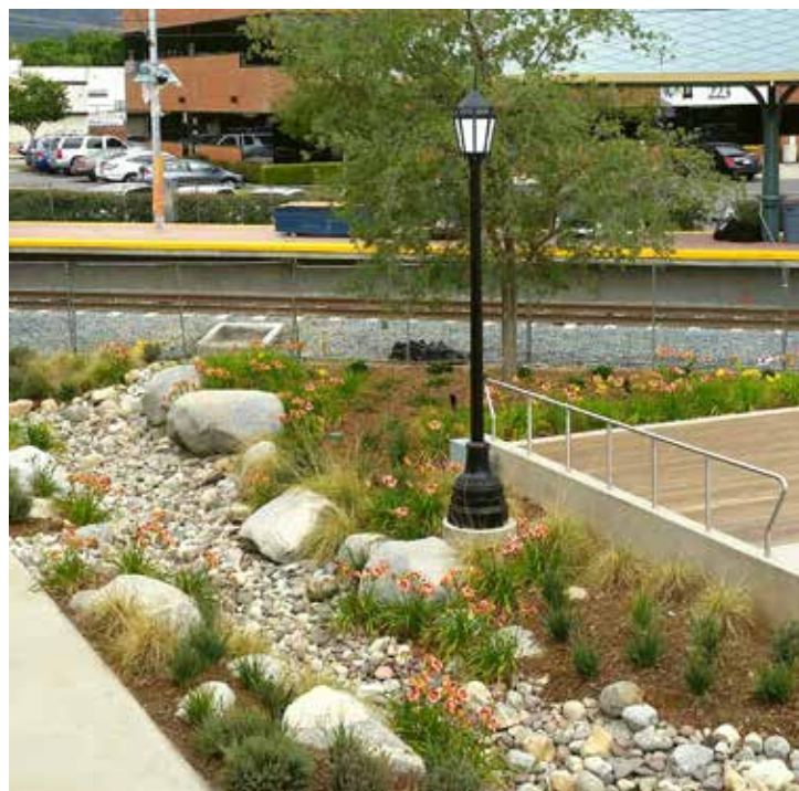
Daylilies and grasses absorb train station runoff.
