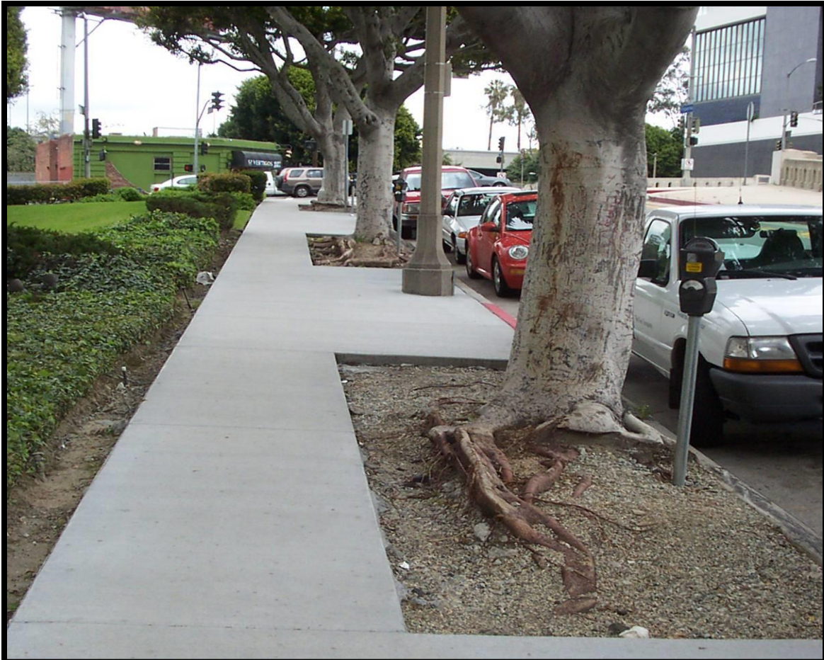
The sidewalk cutout option can be used in some scenarios on downtown streets. The trees are shown before mulch was applied.
