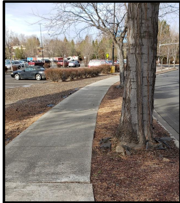
Figure 8 – The additional space available should have allowed greater space between the tree and the sidewalk.
