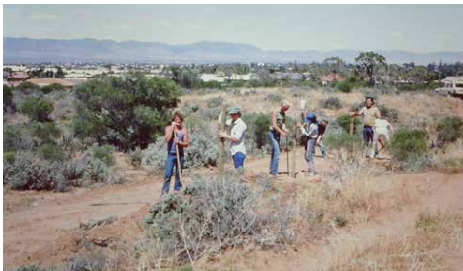
John Brook, far right (bending) working with pastoral industry trainees building the first section of perimeter fencing at the newly acquired AALBG site 1985. Materials were paid for by the Friends.
