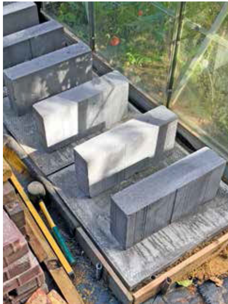
Two blocks per butt were added...
