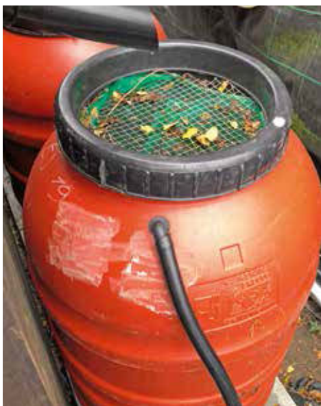
An overflow pipe was attached
