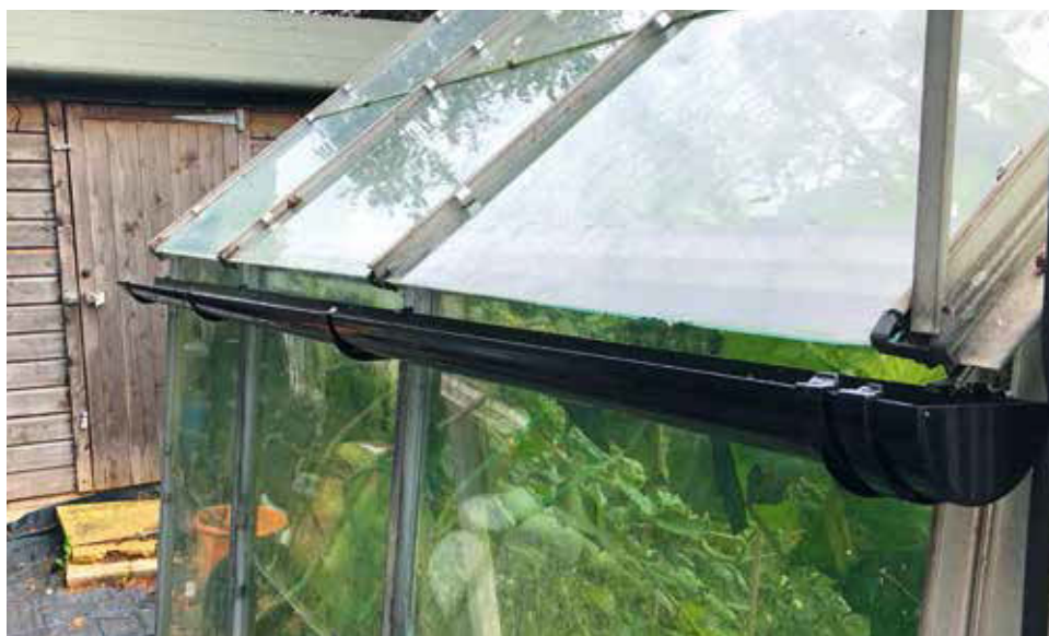
Cable ties were used to connect support brackets to glazing bars on the greenhouse
