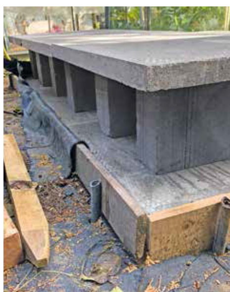
Side view of a completed base
