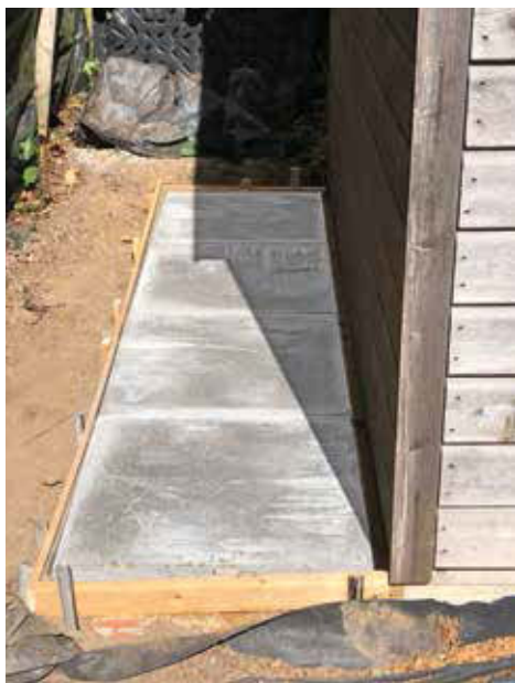
Slabs were laid on top
