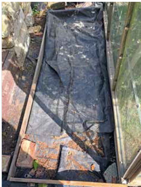
Creating the bases: lining the shuttering
