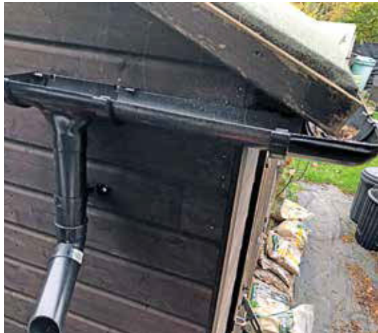
The guttering and downpipe in place
