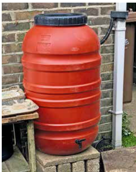
Single butt connected to a downpipe
