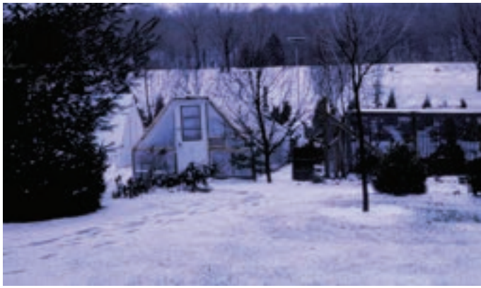
Seen here are the rear of the holding houses and the greenhouse at Lehigh, PA (USDA Zone 6a). The flat-topped holding houses collapsed in a winter rainstorm; one of many rookie mistakes.
