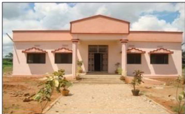
View of Bio-Control Laboratory Building, HRS, Aswaraopet
