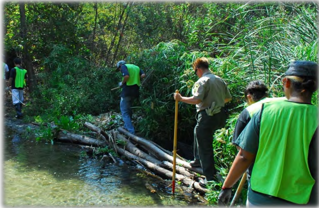
Photo 7. Blocked outflow channel into Haines Canyon Creek.
