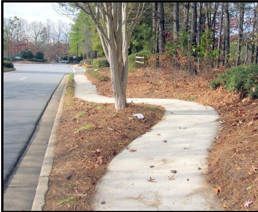
Figure 11 – Re-routing sidewalks around a large tree is a successful option.
