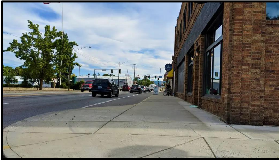
Figure 10 – When designing the tree opening, ask yourself what the minimum size of paving would be instead of the minimum size of the tree opening. Additional space available will help reduce conflicts between roots and paving and improve the soil growing conditions.
