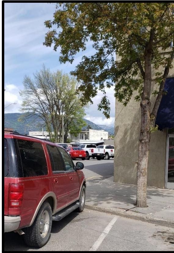
Figure 9 – As trees grow grates girdle trunks and create trip hazards.
