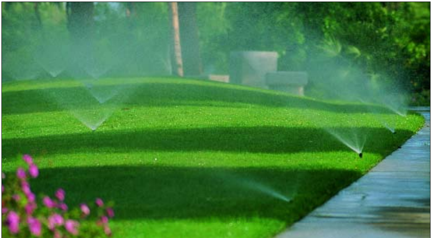
Installed and operated correctly, an automatic sprinkler system is the ideal way to irrigate lawns.
