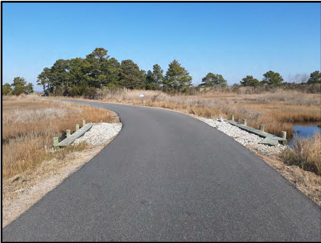
Photograph 6: Roadway culverted stream crossing
