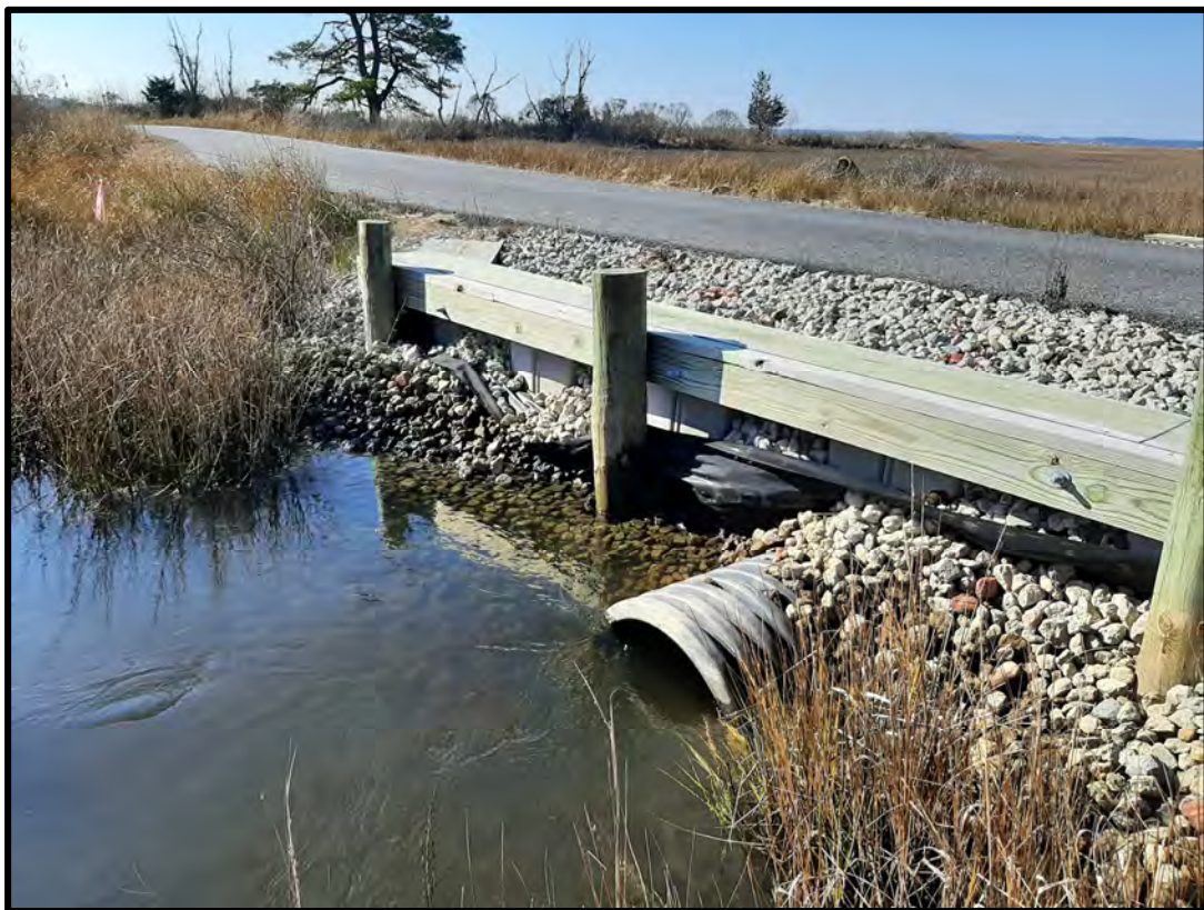
Photograph 8: Eastern side of culverted stream crossing
