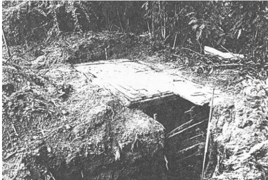
Figure 28: Partly uncovered shelter during repairs. Northern roof and northwestern wall are exposed showing the shaft.
