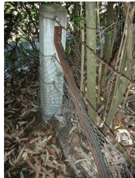
Figure 53: Concrete post and stay.
