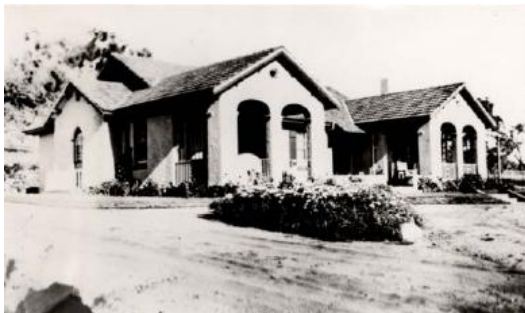
Figure 110: c1930 - Banks grassed, triangular plot planted, planting around house established
