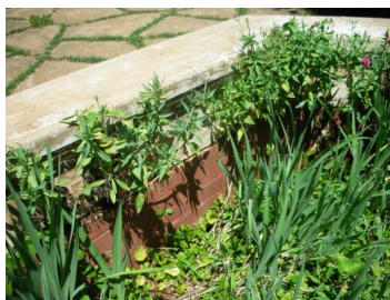
Figure 45: Invasive SSP should be removed from entry wall.
