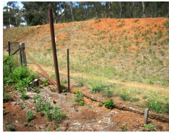
Figure 60: Cast iron post and timber at rear boundary.
