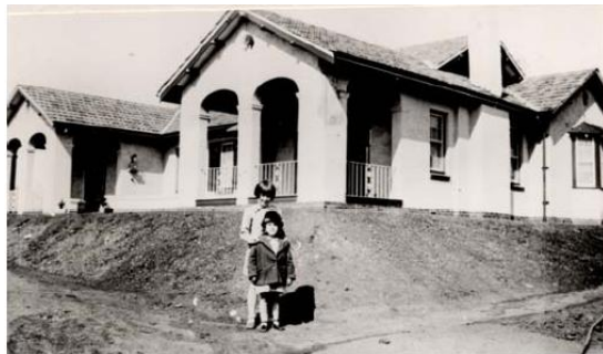
Figure 103: Mid 1927 – Earth banks not grassed, though hoses being used to water side garden
