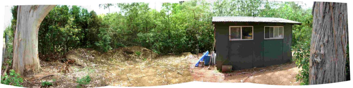
V48: Back Shed
