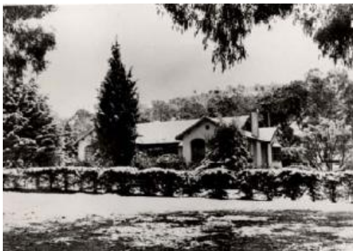
Figure 117: 19 July 1949 - Hedge providing some screening, cypresses approaching maturity. Golden cypresses continue to grow and destroyed original scale and design intent of the garden.
