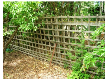
Figure 63: Part of 1980s reconstructed fence to north orchard.
