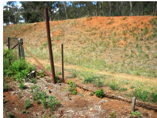
V33: Cast iron post and timber at rear boundary.
