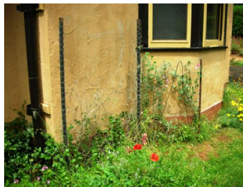
Figure 62: Existing sweet pea frame.
