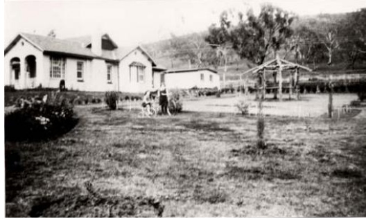
Figure 107: Early 1929 – Climbing roses evident on arbour, rectangular lawn manicured, surrounding area slated to be later developed into shrubbery, hedges established separating vegetable garden with an open paling fence across block behind garage
