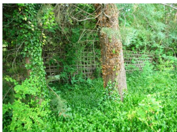
Figure 42: 1980s lattice fence under assault from various weeds.
