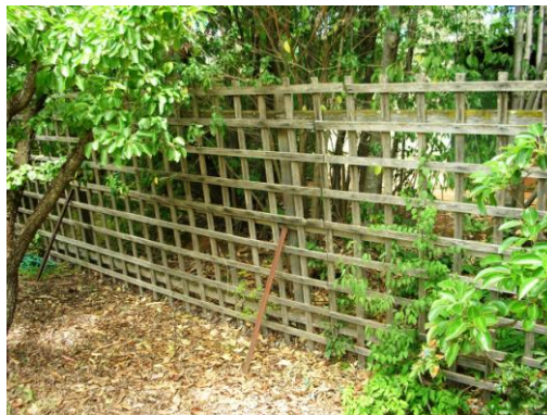
V36: Part of 1980's reconstructed fence to N orchard.
