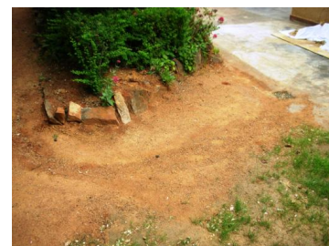
Figure 65: Runoff near the gravel drive needs monitoring and the drain cleared.
