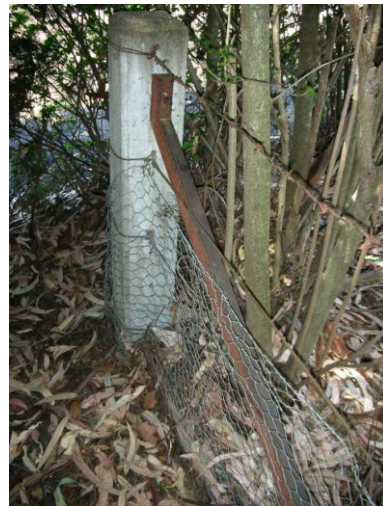
V26: Concrete post and stay.
