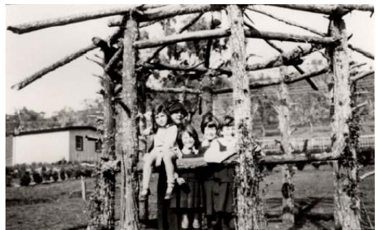
Figure 106: Spring 1928 – detail of arbour, new hedges and paling fence.
