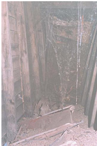
Figure 30: Interior as found, facing north (26 March 1990)
