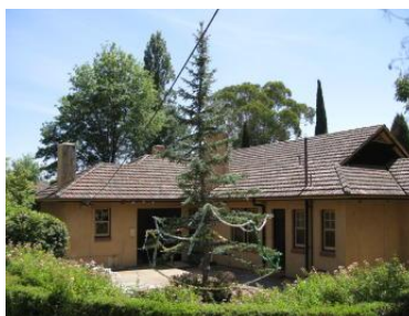
Figure 82: Rear, south west
