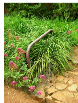
Figure 47: Existing intrusive handrail needs to be replaced.
