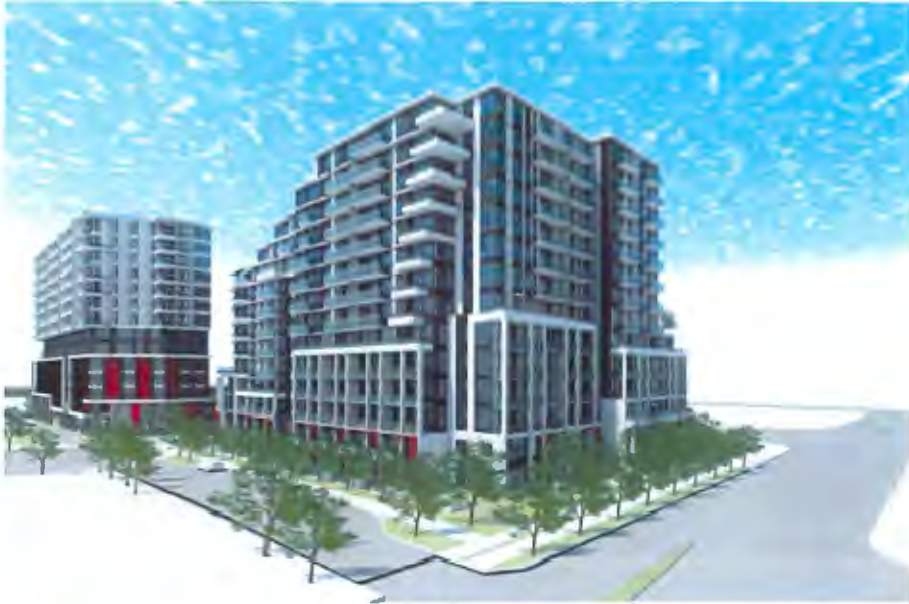
VIEW TO BUILDING J (PHASE 3) FROM SOUTHEAST
