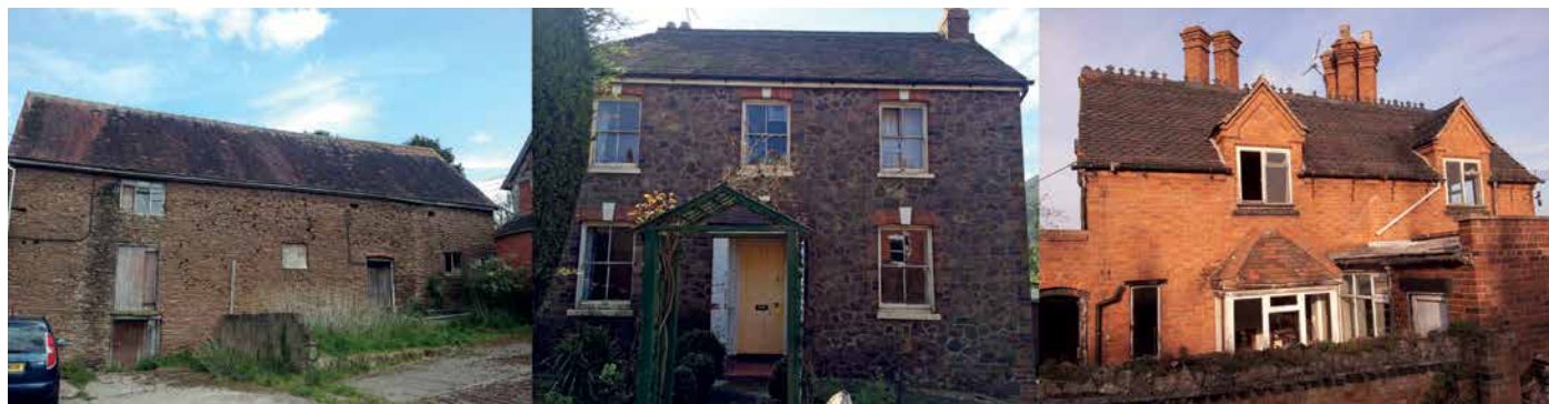
Figure 1. Buildings assigned low, moderate and high roost suitability – which is which? Initial impressions are not always accurate.
