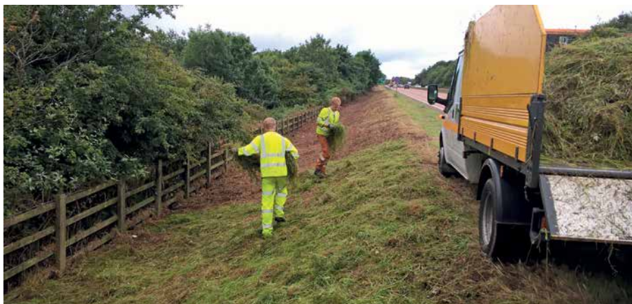
Figure 6. Spreading seed material (green hay) on prepared ground along the road verge. The use of additional, locally sourced wildflower seeds can also be used as part of this process. Photo credit Leonardo Gubert.
