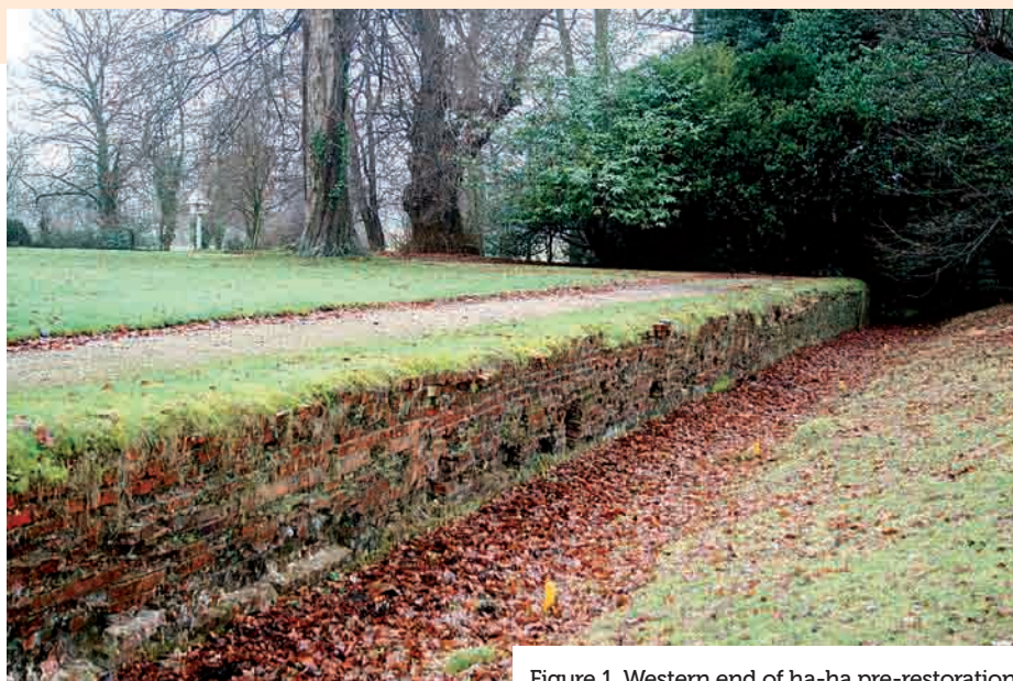
Figure 1. Western end of ha-ha pre-restoration.
