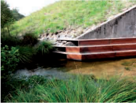
Figure 3. Semi-aquatic mammal ledges at a range of heights to adapt to changes in seasonal water levels. These are integrated with the surrounding habitat.
