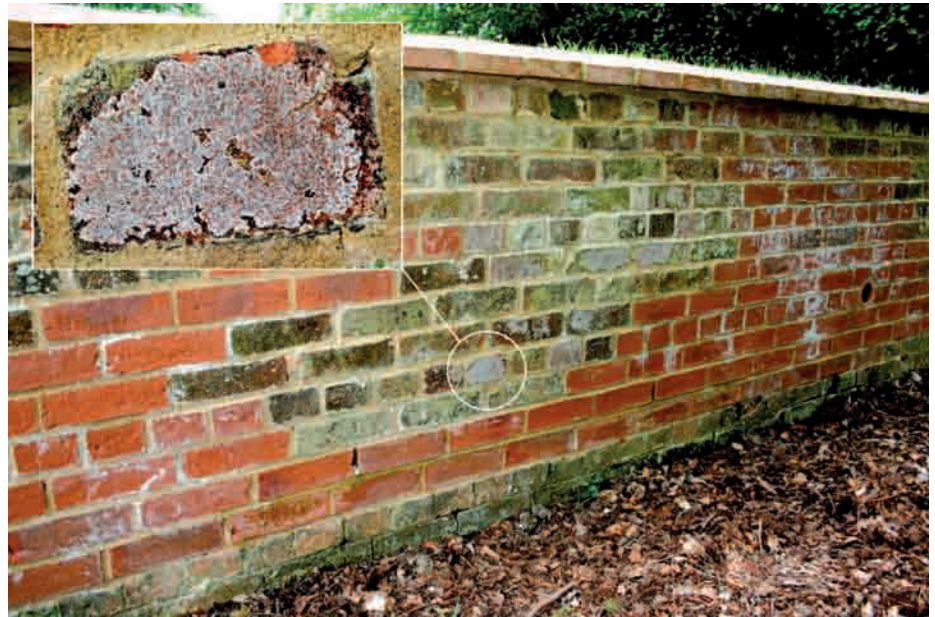
Figure 4. Marker thallus (circled) one-year post-restoration. Inset shows close up of marker thallus.
