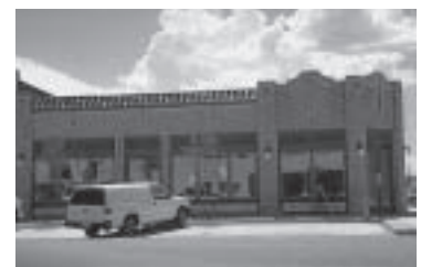
A building's mass and scale can be modified using pilasters, parapet details and changes in materials.
