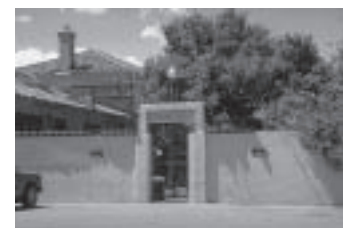
Architecturally compatible screening of outdoor dining.
