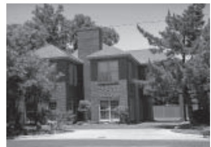
This new structure is large, but the form is articulated like a residential building in terms of form, detail and roof shape.
