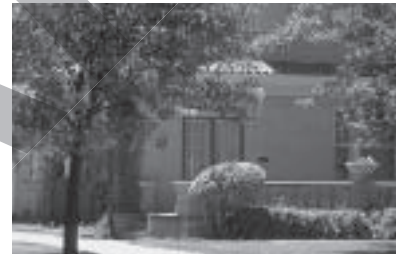
Building materials are typically brick with stone, brick or wood trim.
