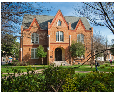
Steeper pitches are appropriate, like that of Tuomey Hall, in Gothic Revival buildings including those around the Woods Hall Quad.
