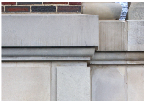
Above: Water table is sloped to shed water and protect stonework below.
