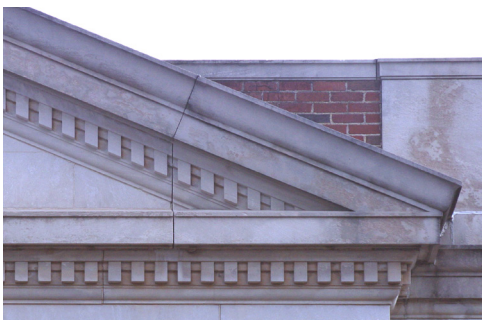
A product of the pitched roof design is the tympanum or triangular pediment at the gable end. Where it occurs, this element is part of the crown. The tympanum is surrounded by projections of the cornice profiles.
