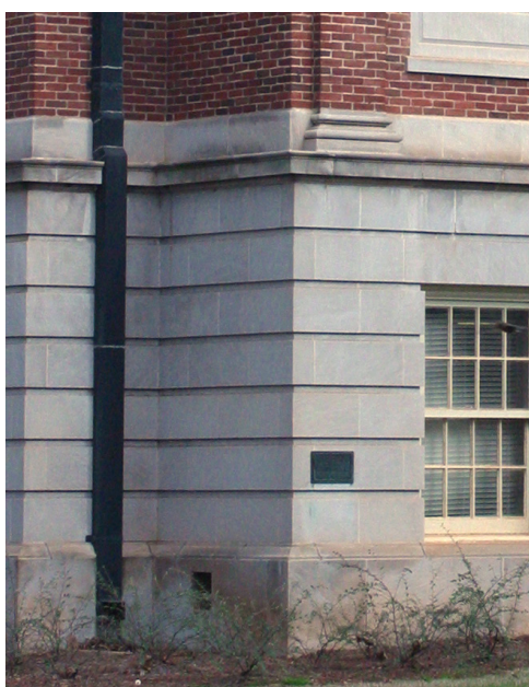
Above: Base projecting outward from the shaft.
