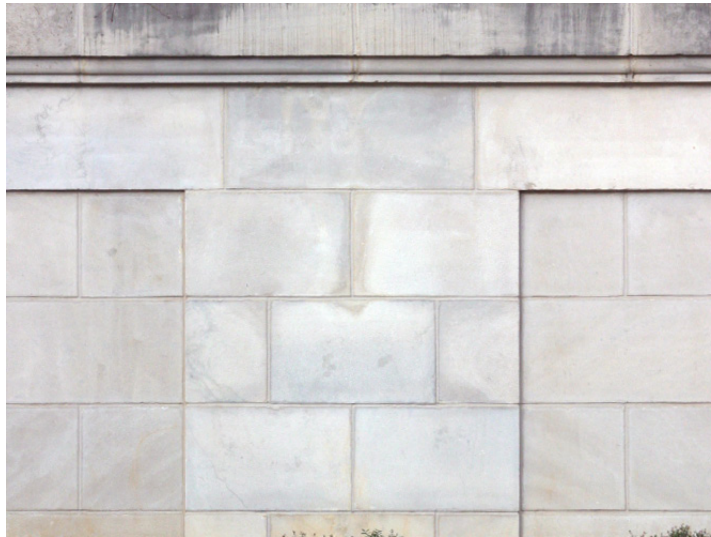
Campus buildings have used detailing to enhance the monumental nature of their bases through exaggerated joints and panel size.
