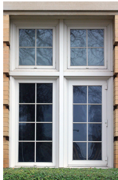
Above: Historic example of the stacked window design
