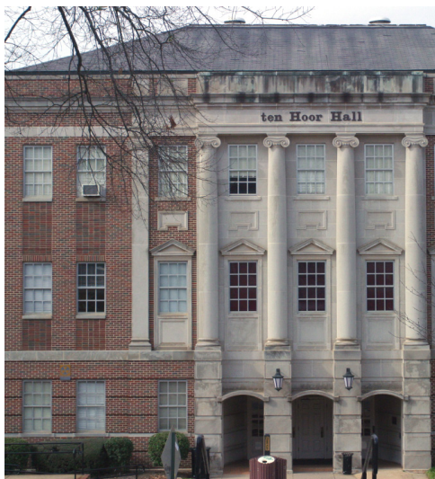
Campus buildings use classical architectural elements, such as columns that span two stories, vertical openings, and extruding building volumes to accentuate verticality in otherwise horizontal building masses.
