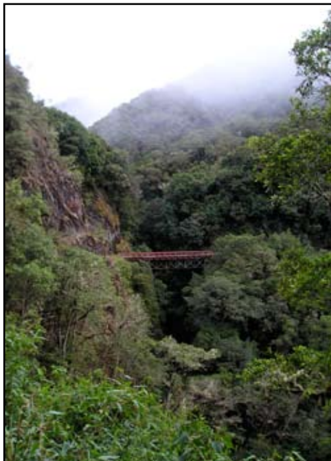
Bridge to nowhere
