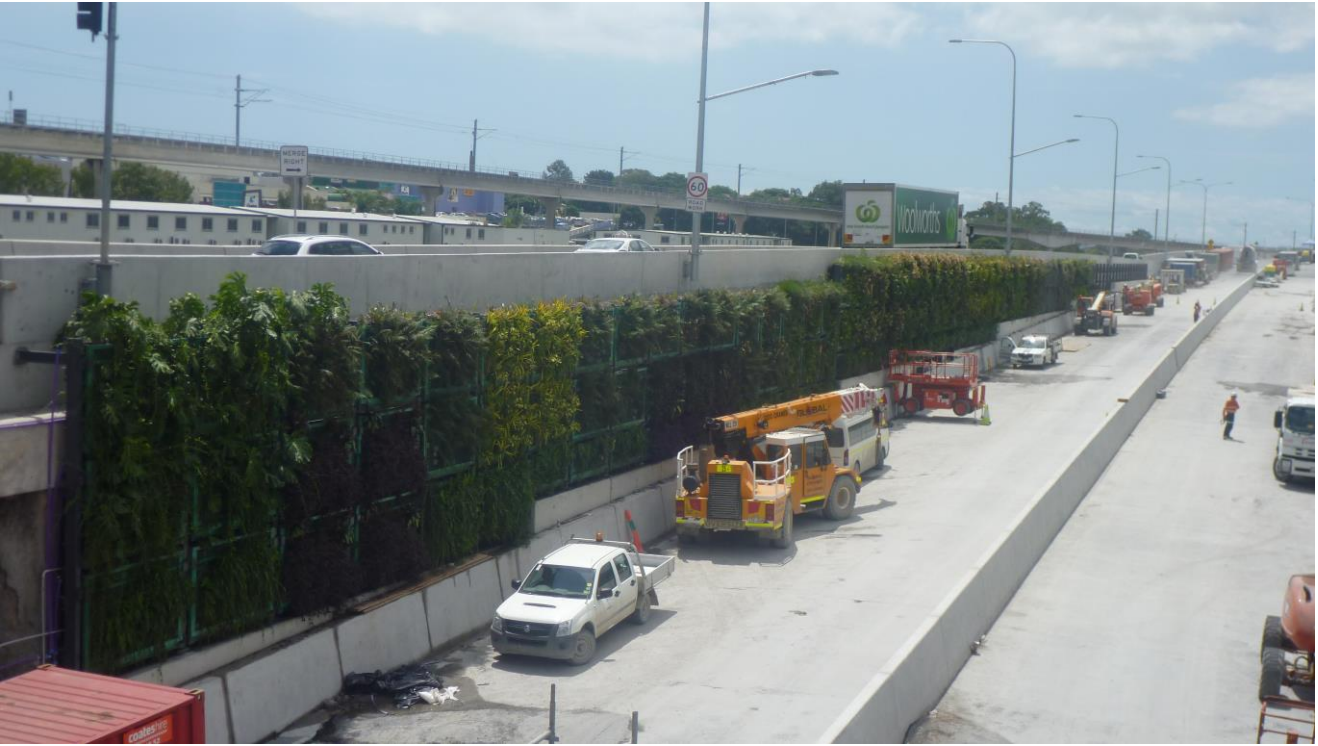
Photo 1a. Airport Link Green Wall under construction
