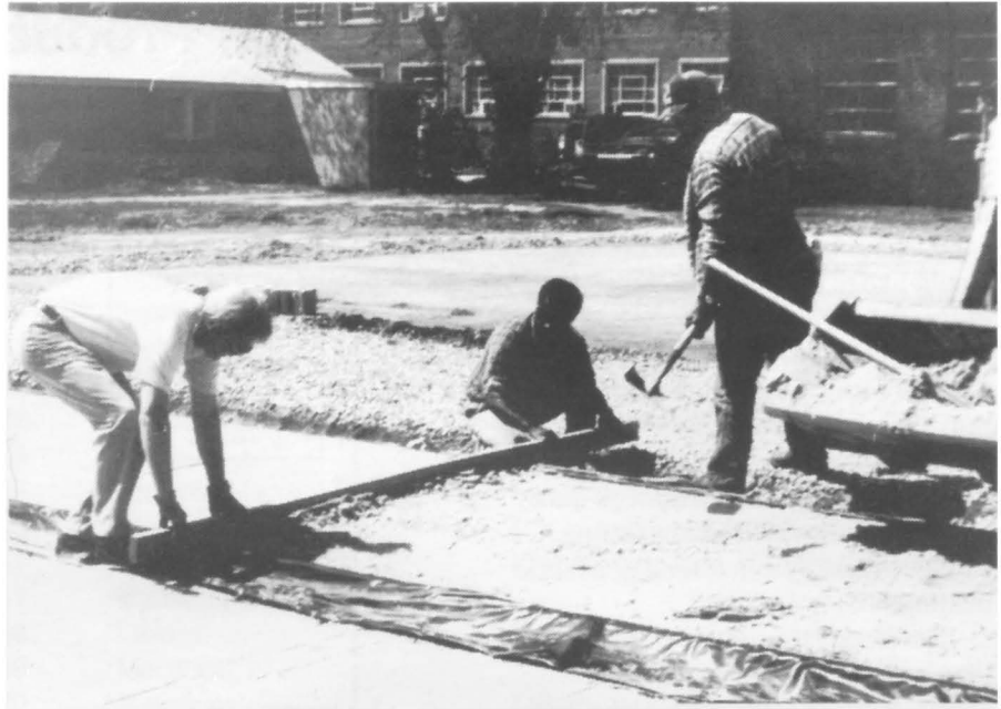
Leveling the sand surface following construction of the capillary beds
