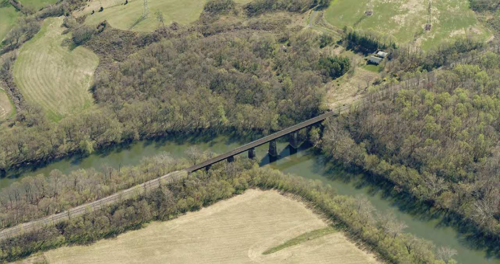
Railroad bridge north of the Monocacy Aqueduct
