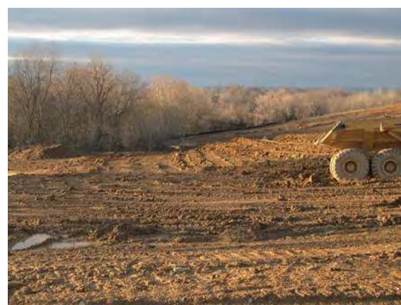
Mass grading for land development
