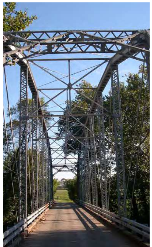
Bullfrog Road Bridge over the Monocacy River
