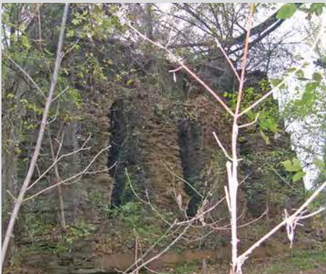
(2) Remnants of Jug Bridge abutment.
