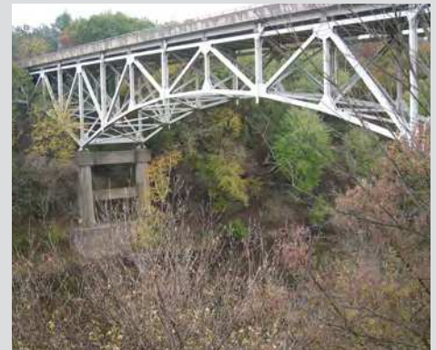
(4) Current truss bridge.
