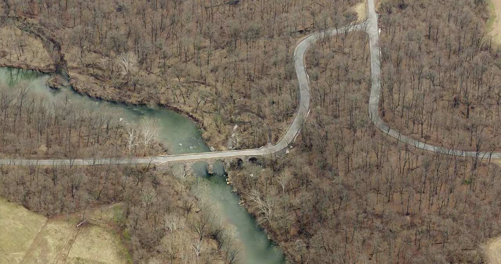
Aerial View of LeGore Bridge
