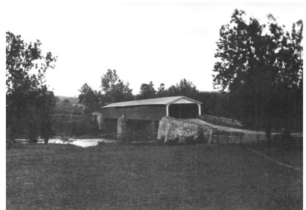
19th Century bridge over the Monocacy near present day MD355.
