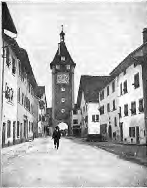
Neunkirch. (C. Schaffhouse). L'Oberthorthurm.
