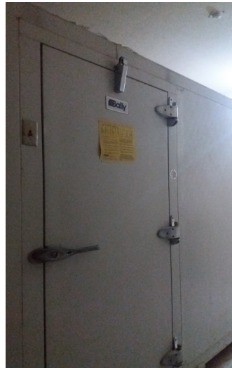
Plate 6. Cool room of Postharvest Division, BARI (Temp. 6.5 to 7.5 o c, Humidity 70 to 75%)
