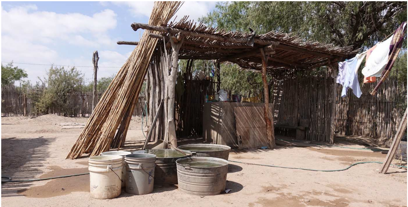
Figure 4. Ramada for washing, Pótam. Vaaka poles, roofing, and fence; corner post is cottonwood ( Populus mexicana subsp. dimorpha ). Photo by Peter Blystone, 1 Jun 2019.
