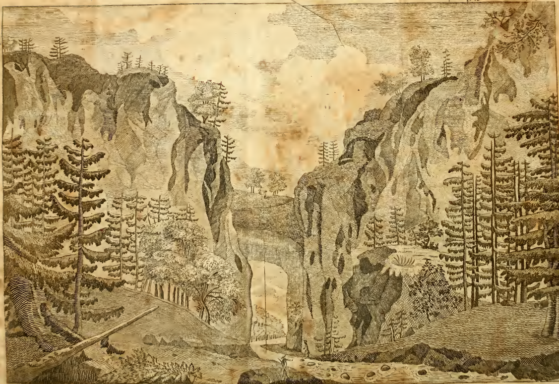
A View of the Natural Bridge in Virginia.
