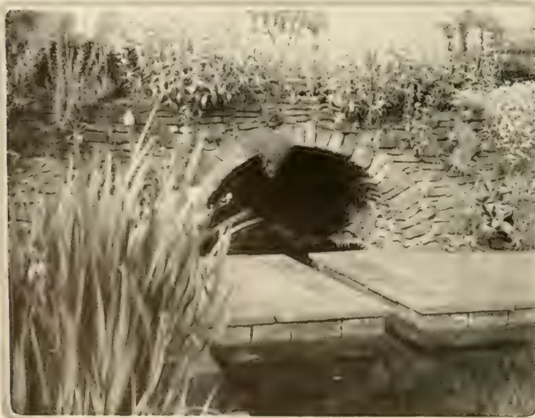
The arch forming the inlet to the water parterre, in the illustration below this, is built in dry stone. The treatment of the curb, which is edged with flag-stones, should be noted, since it avoids a too sharp edge in an ingenious manner
