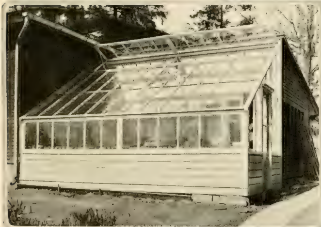
A simple type of lean-to greenhouse, showing the proper type of ventilator. For best results, the lean-to should be heated at night and on cold, cloudy day
