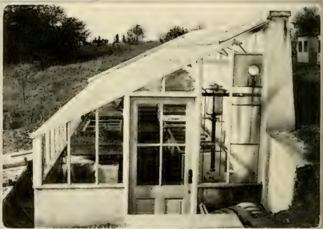
The lean-to above is built against a concrete wall. It is partly sunken and faces the south, to catch and hold the maximum amount of sun warmth
