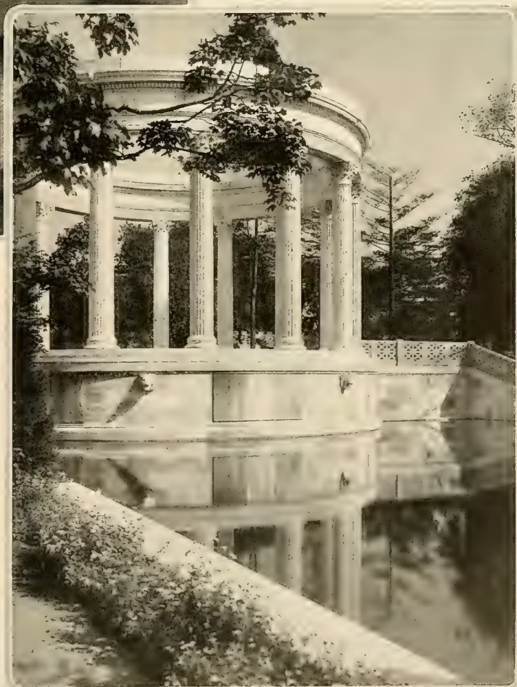
Standing at the edge of the upper terrace and overlooking the swimming pool is a Greek temple of marble Corinthian columns and a circular entablature open to the sky. It is executed in Alabama marble. The whole garden answers the poet's question, "Why Go To Greece?"
