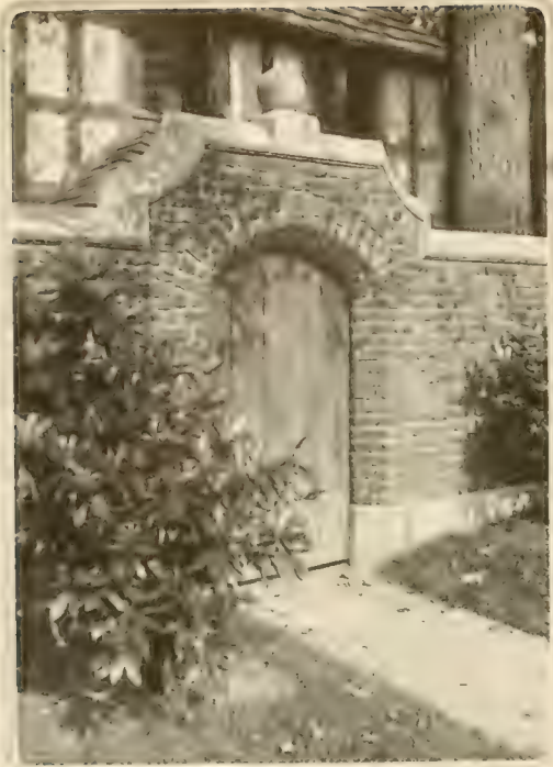
If the garden is walled, the gate can be of solid planks bolted together, which will be in keeping with the rugged character of the brick wall. John Russell Pope, architect
