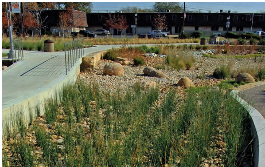
The water detention system at The Green at College Park at the University of Texas at Arlington prevents stormwater runoff from flooding a nearby creek and cleanses it for reuse.
