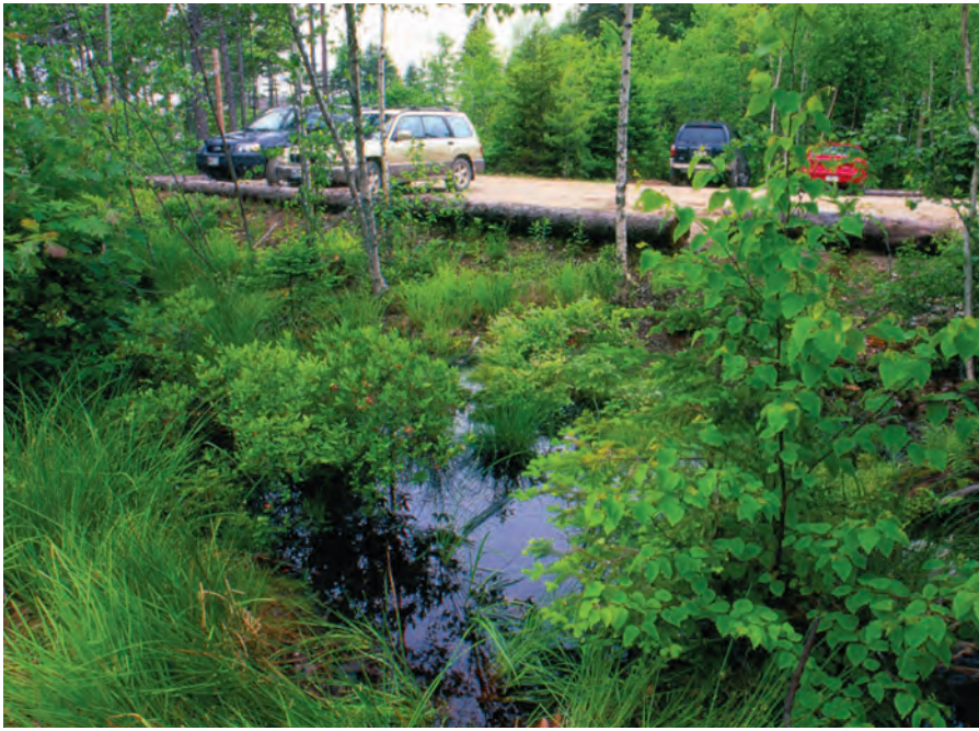
The low-tech gravel parking lots at Coastal Maine Botanical Gardens are separated by naturalistic boggy areas designed to absorb runoff.
