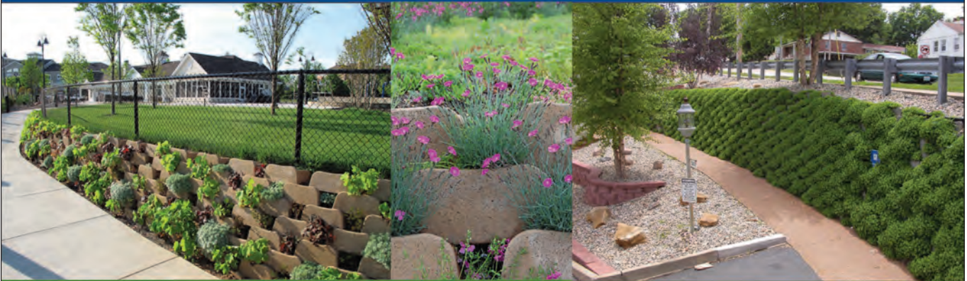
Vertical Gardens/Vegetated Retaining Walls
